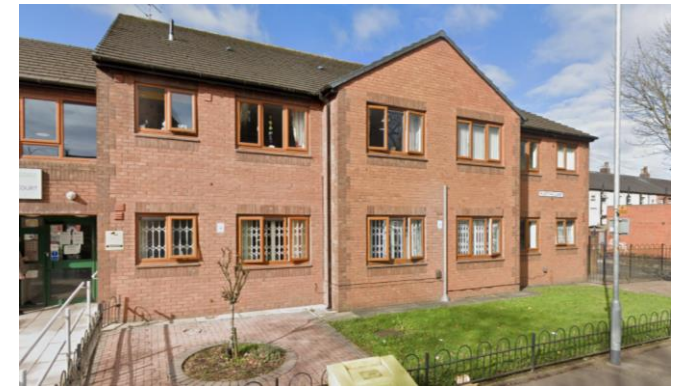
Arnold Bagnell Court Platting Lane
