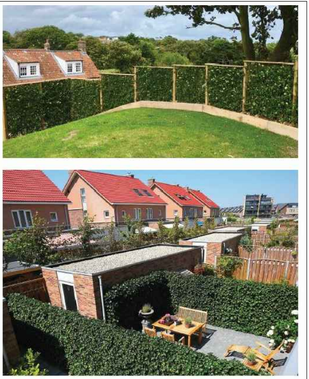
Boundary detail B - Mobile Green Screen ready made green screen system - 1.2m wide panels x 2.2m high planted with Hedra helix 'Woerner'.
