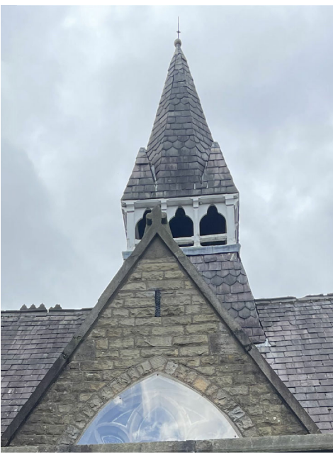
Cupola woodwork undamaged; requires further inspection
