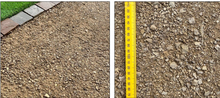
Example images of compacted gravel.
