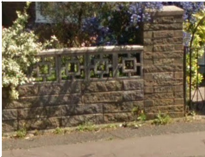
front boundary wall
