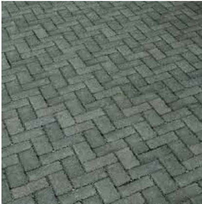
M3 Driveway / Access Road Surface
