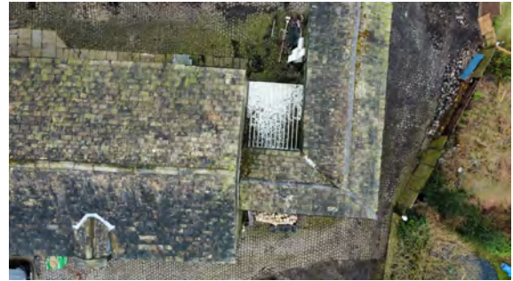
Image 5 - General condition of roof tiles on B1.
