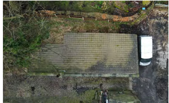
Image 6 - General condition of roof tiles on B2.
