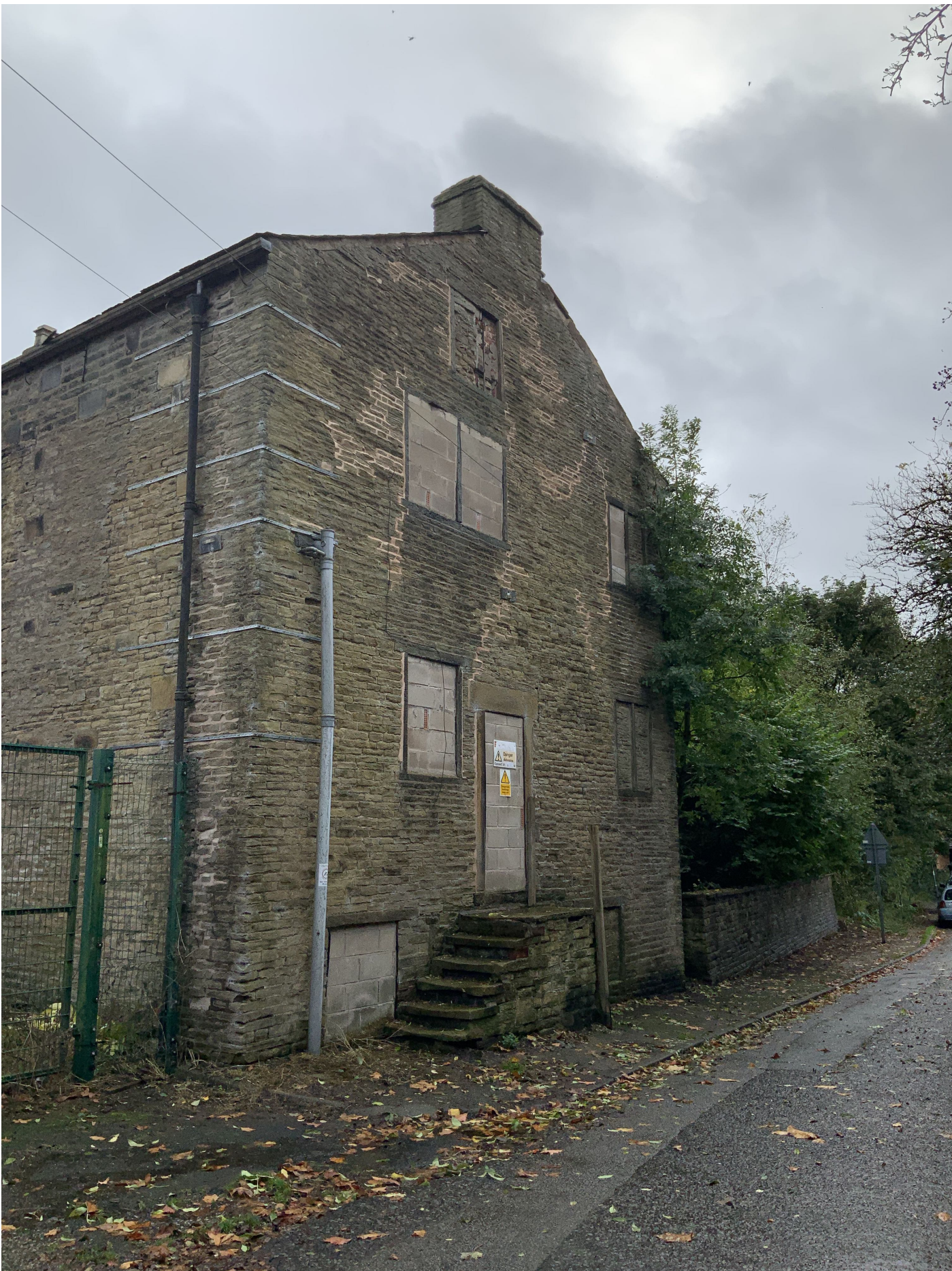
NORTH WEST GABLE
