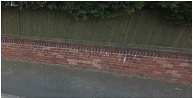
ADJACENT BOUNDARY WALL.
