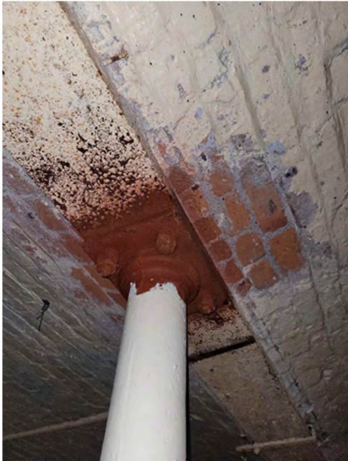
03 Column Type 02 - Sample Image of Existing n.t.s @ A1
