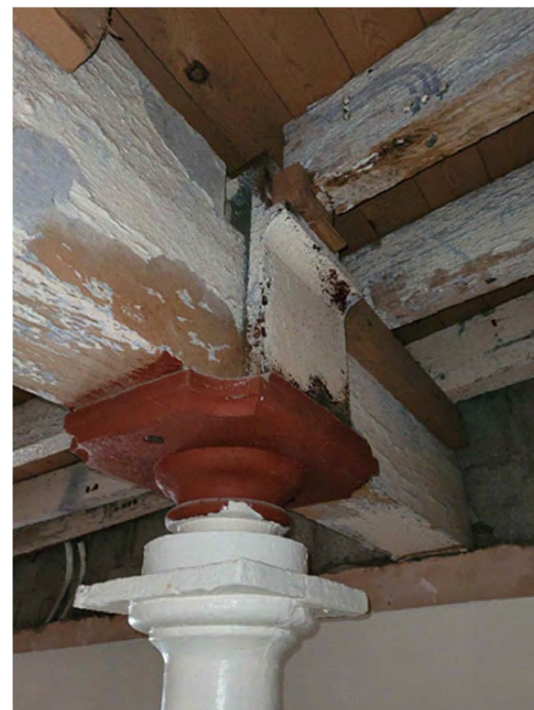
03 Column Type 01 - Sample Image of Existing 0001 n.t.s @ A1
