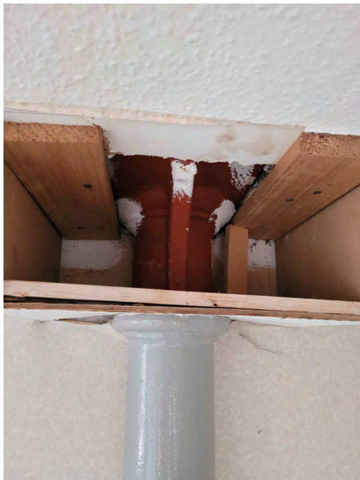
03 Column Type 08 - Sample Image of Existing 0001 n.t.s
