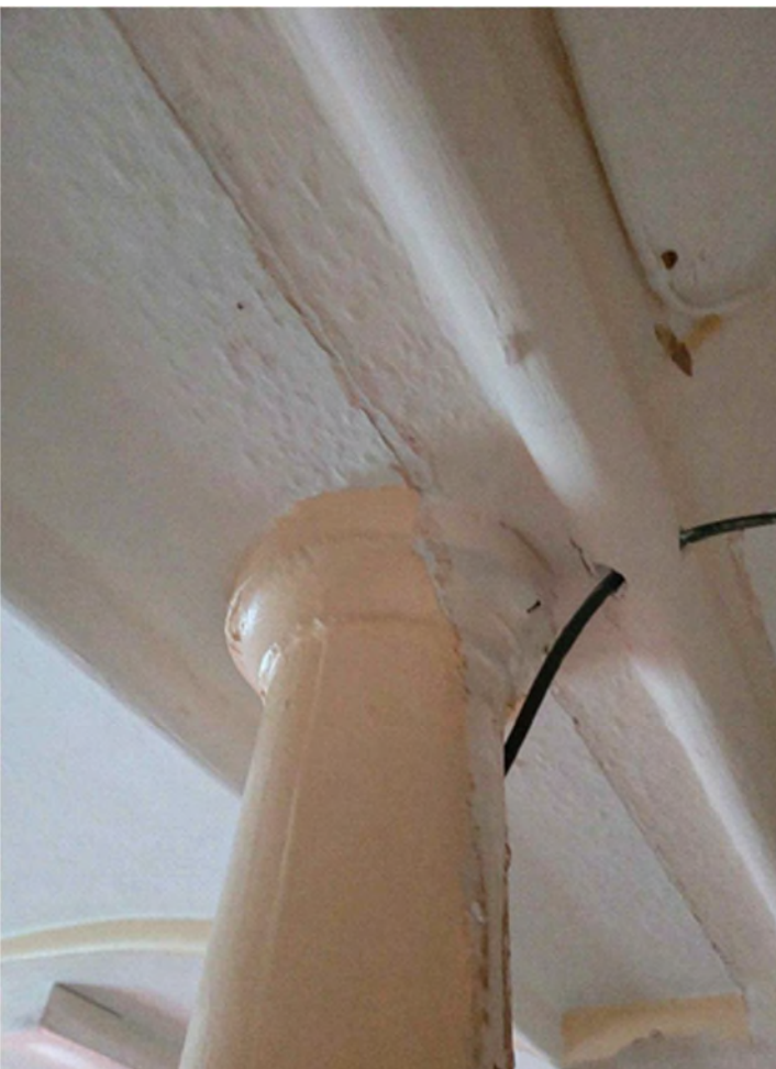
03 0001 Column Type 05a - Sample Image of Existing (Refer to Schedule for individual images) n.t.s @ A1
