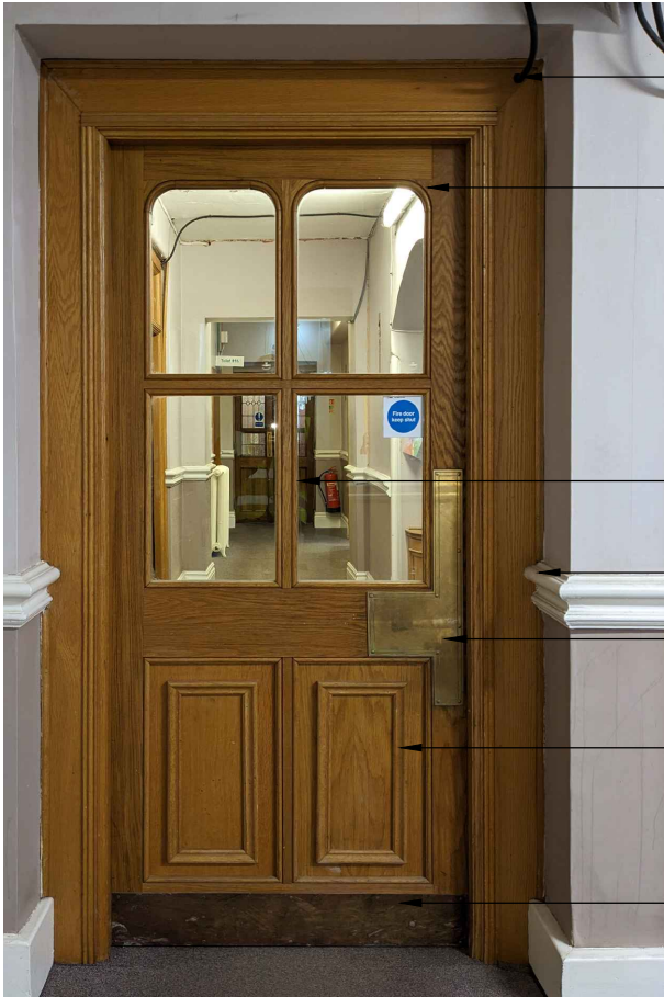
EXISTING VIEW OF DG13a.3 FROM G13.a SIDE
