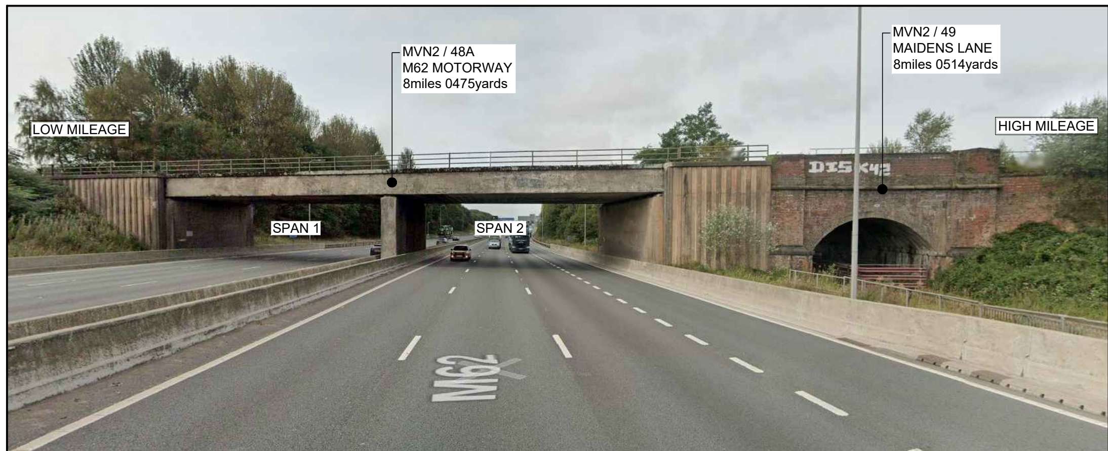
EAST ELEVATION (UPSIDE) FROM M62 MOTORWAY
