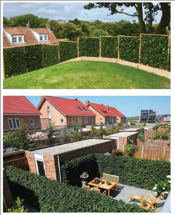
Boundary detail B - Mobilane Green Screen ready made green screen system - 1.2m wide panels x 2.2m high planted with Hedra helix 'Woerner'.
