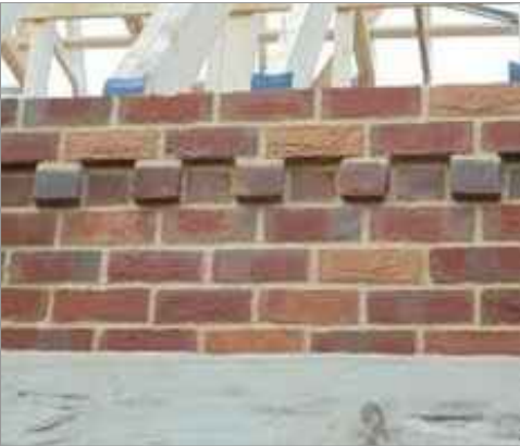
Eaves brick corbel detail -Butterley carbon black rustic
