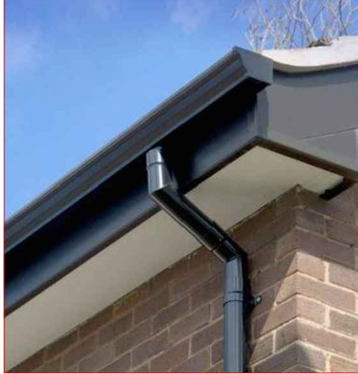
Seamless aluminum gutters and downpipes finished in black
