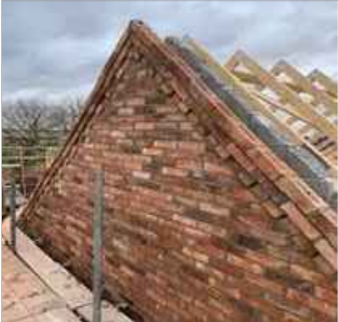
Verge brick corbel detail - Butterley carbon black rustic
