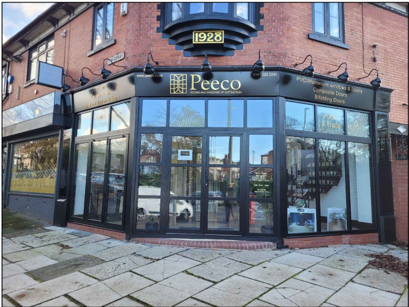
Photo - With New Shop Front Installation
