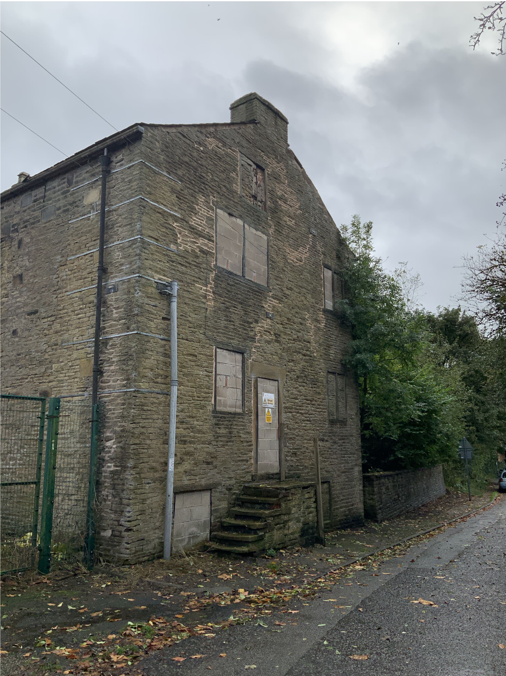
NORTH WEST GABLE
