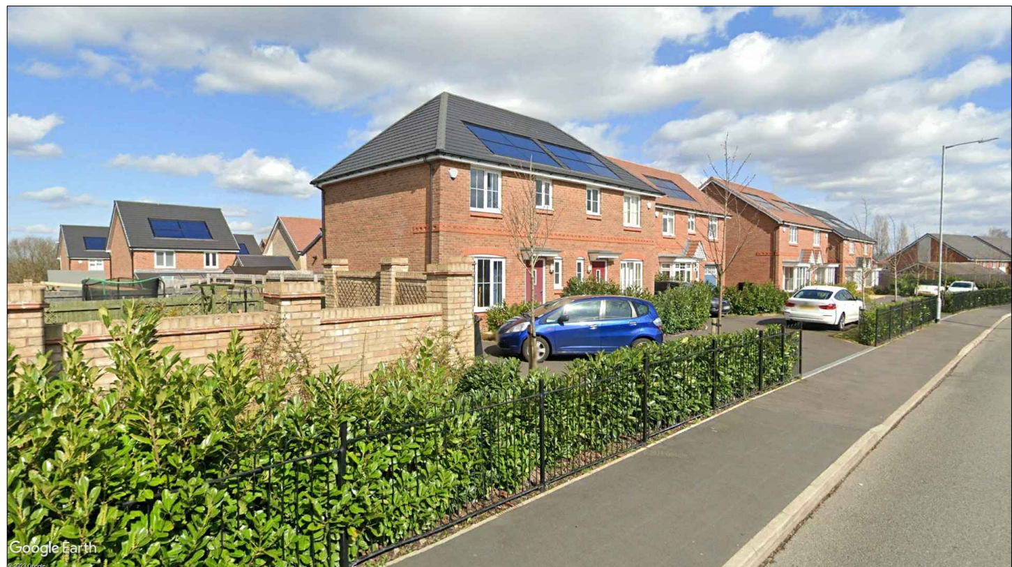
PHOTOGRAPH 3 - EXAMPLE OF FRONT & REAR PV PANELS (DETACHED & SEMI DETACHED)
