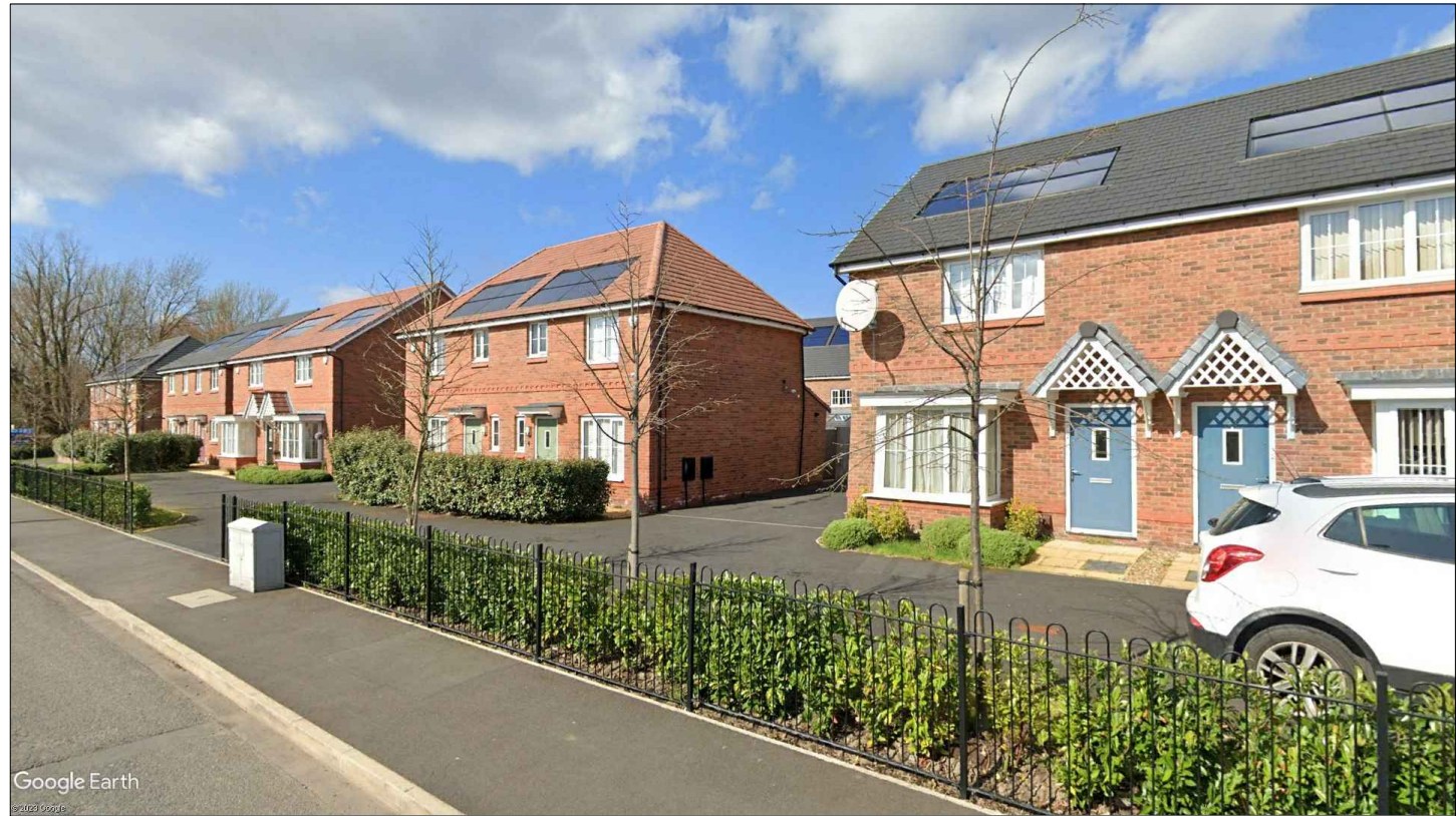
PHOTOGRAPH 2 - EXAMPLE OF FRONT PV PANELS (SEMI DETACHED)
