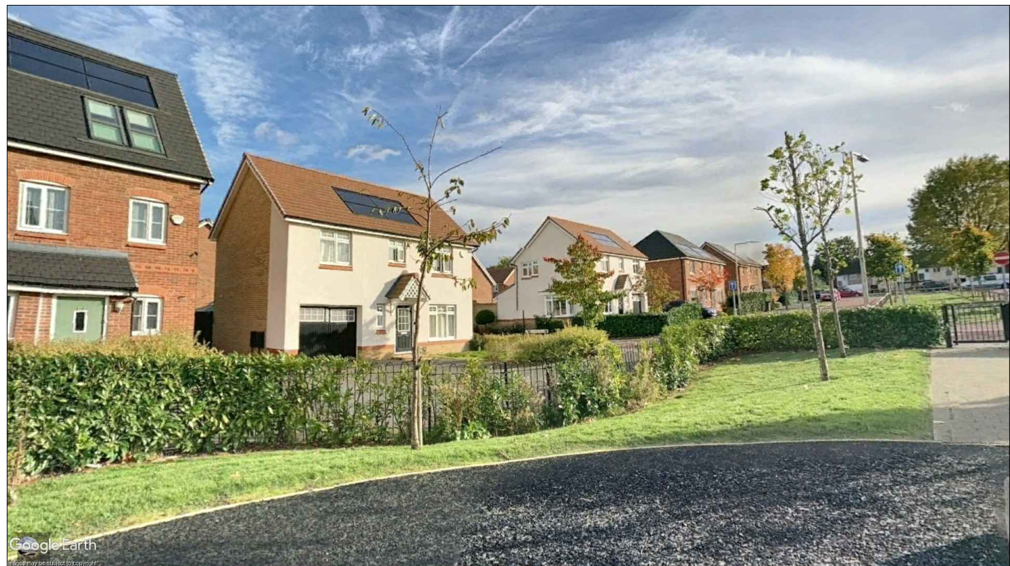
PHOTOGRAPH 4 - EXAMPLE OF FRONT PV PANELS (DETACHED & 2.5 SEMI DETACHED)
