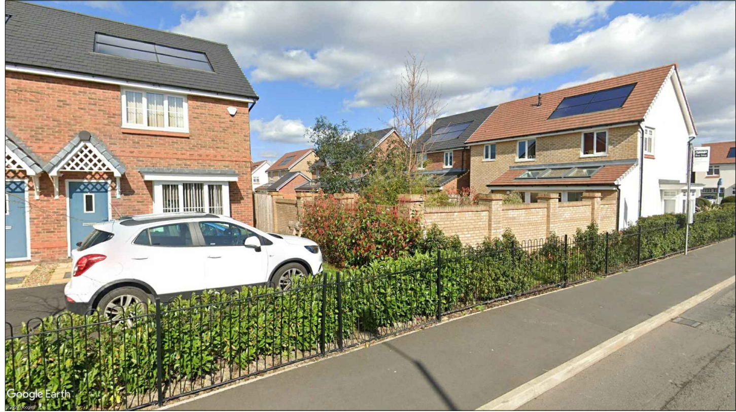
PHOTOGRAPH 1 - EXAMPLE OF FRONT & REAR PV PANELS (DETACHED & SEMI DETACHED)
