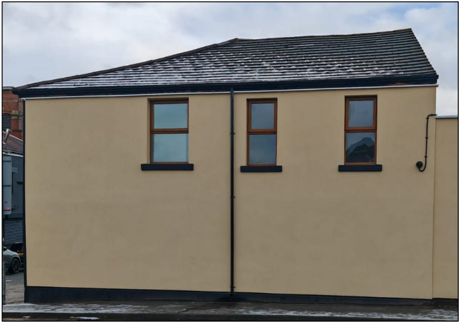
67 Whitehall Street,Rochdale showing newly profiled cills. (Courtesy of RS Rendering Ltd.)
