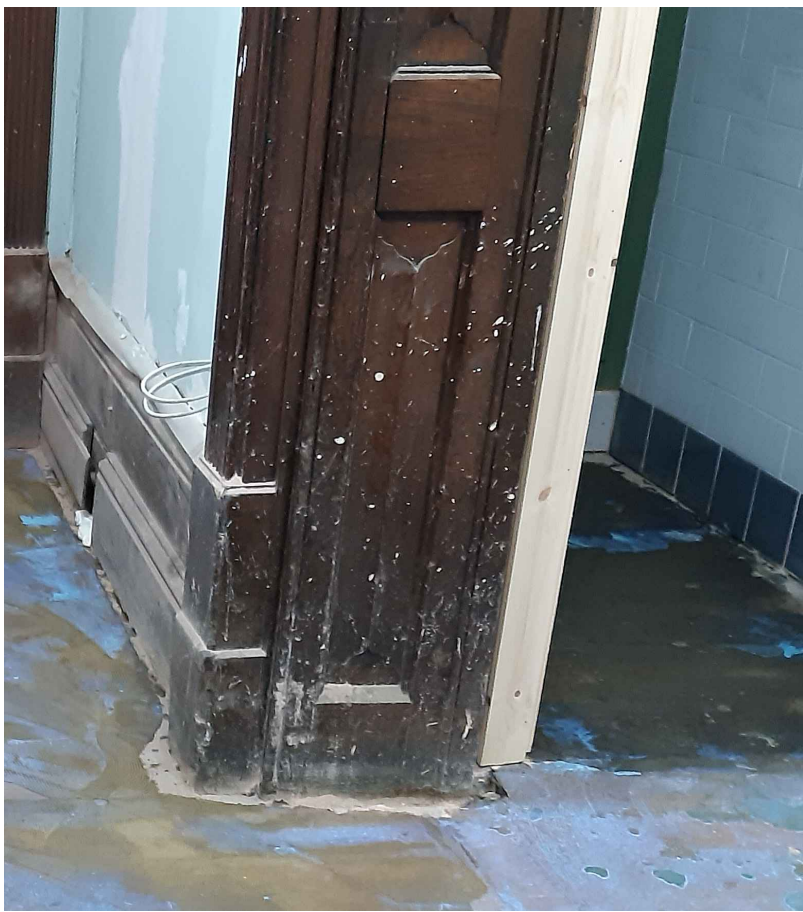
2no. cupboard door panels to reflect existing adjacent door lining panels on site.
