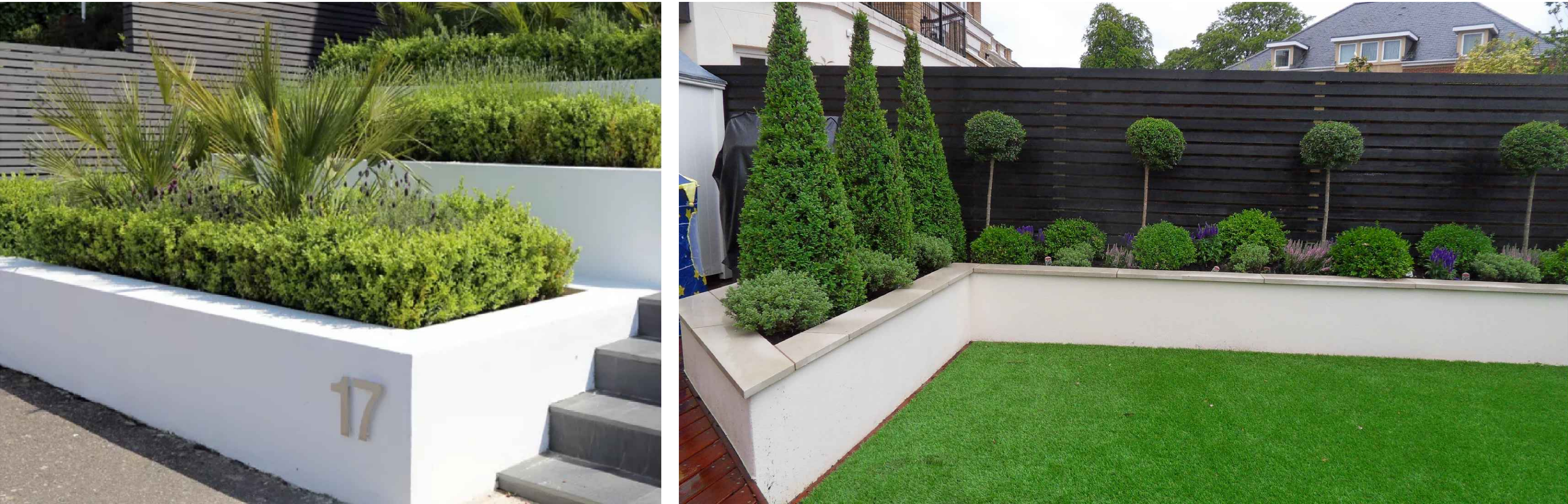
Retaining wall B - Brick retaining wall within gardens. ■
