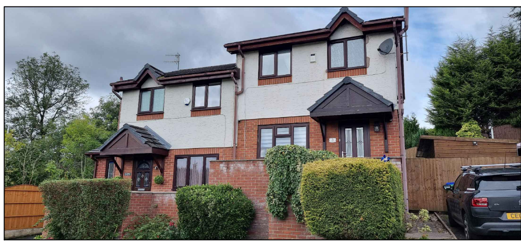
Site Photo-Existing Front Elevation (N.T.S)
