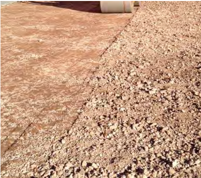
Compacted MOT Type 1 aggregate
