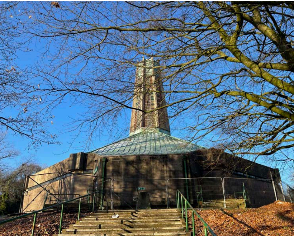
9 View from the existing stepped access up the hill towards the building from the South-West
