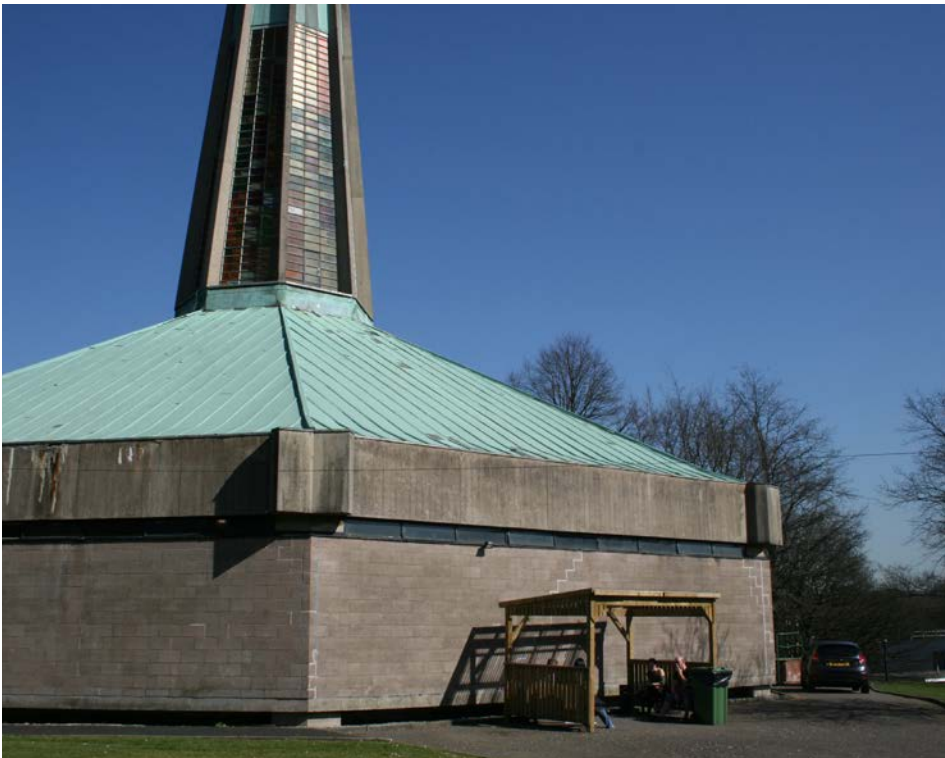
10 View onto the existing parking area to the south.
