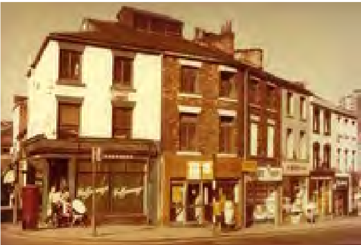
Figure 104: A 1981 photograph of Drake Street, showing 8 Drake Street to be exposed brick but with its windows replaced on the first and second floors and a c.1970s asymmetrical shopfront with a deep fascia (Source: Anstess 1981b).
