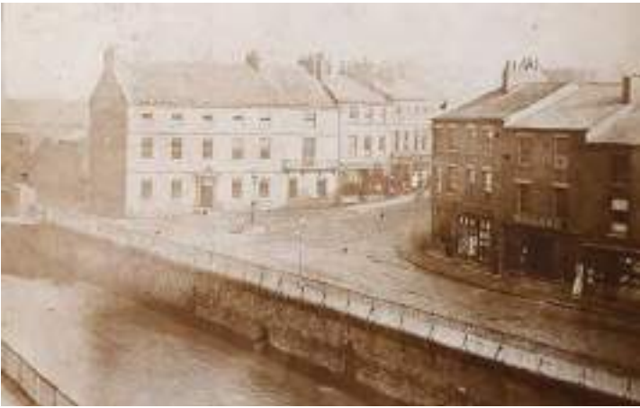
Figure 42: The earliest photograph obtained of the property, dating to c.1855, showing the corner of Drake Street and South Parade, showing the eastern end of the front elevation of 9-10 South Parade which was likely to have comprised a three-bayed three-storey Georgian terraced building with exposed brickwork, timber framed double-hung sash windows and a slate tile roof, with a ground floor mid-19th century symmetrical timber-framed shopfront on the ground floor (Source: TR Dig Streets 545).
