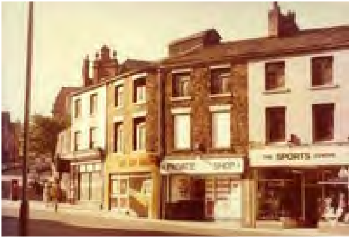
Figure 110: A 1981 photograph of Drake Street, showing 10 Drake Street with exposed brickwork and the windows on the first and second floor elevations to have been replaced in the 1970s. The shopfront appears to be a 1970s tiled shopfront with aluminium-framed glass (Source: Anstess 1981a).
