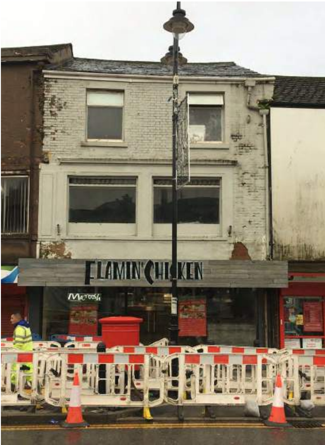
Figure 54: A current photograph of 11 South Parade (Source: Purcell 2019).
