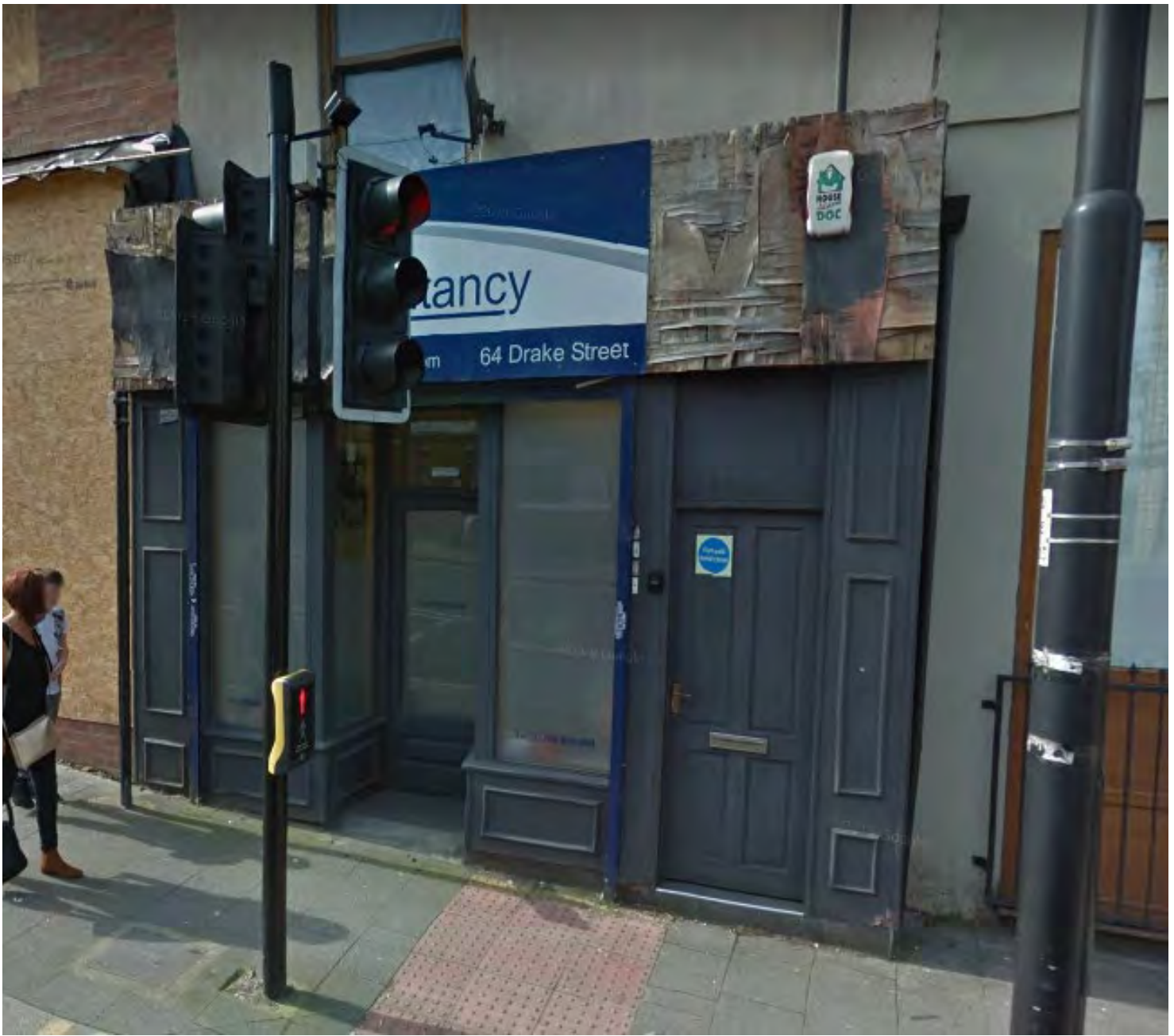
Figure 23: 64 Drake Street, showing a modern interpretation of a historic shopfront, with timber panelled pilasters and stallrisers, a recessed entrance and a timber-framed door with a fanlight above, but with an unsympathetic deep fascia made from poor materials and frosted glass panes (Source: Google 2018).
