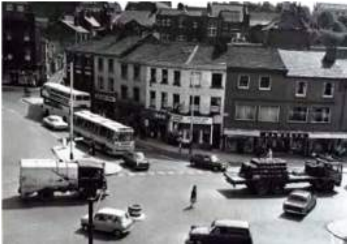
Figure 62: A 1966/67 photograph of Drake Street and South Parade, showing 11 South Parade occupied by Haworth on the ground floor, with altered first-floor windows and replaced frames in the second floor (Source: Rochdale Local Studies 1966/67).
