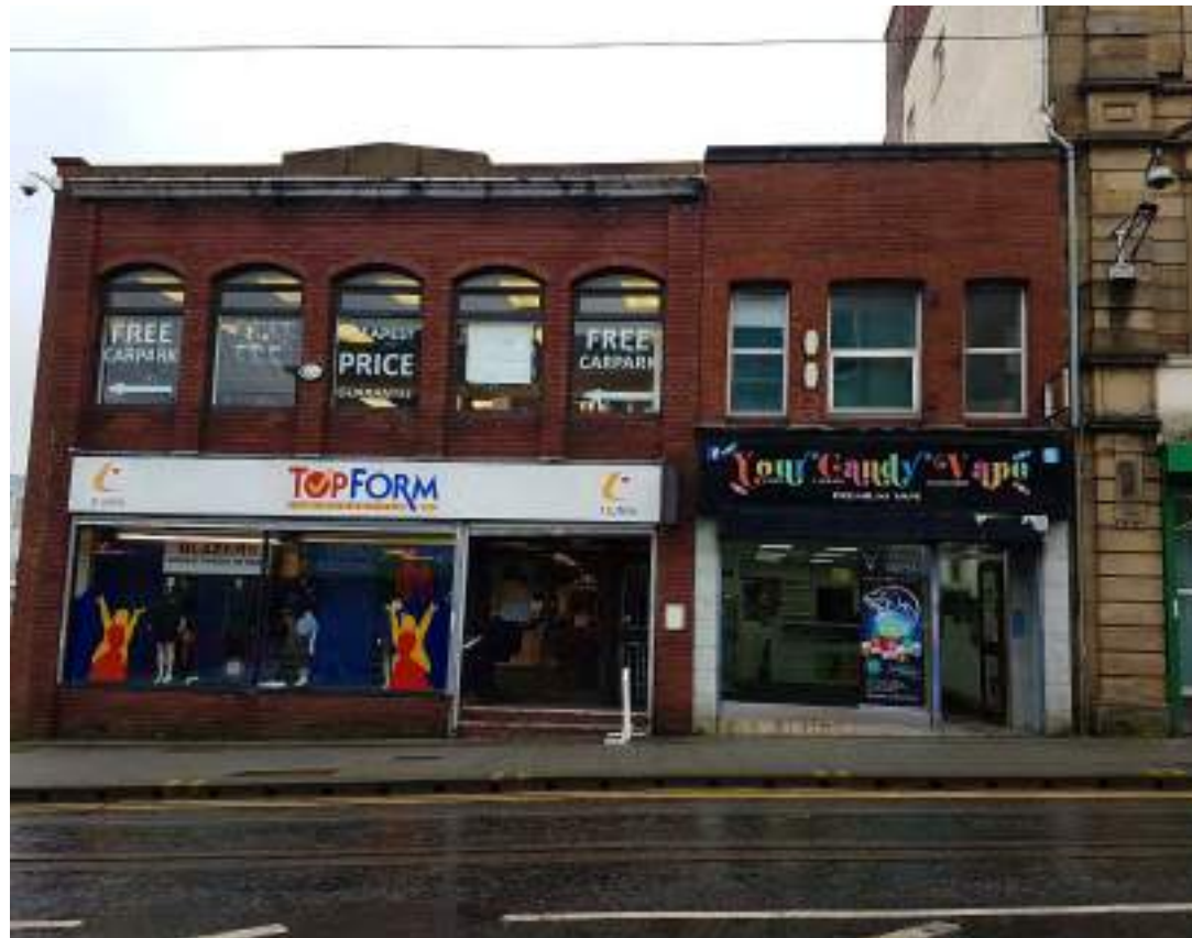
Figure 122: A current photograph of 55 Drake Street (Source: Purcell 2019).
