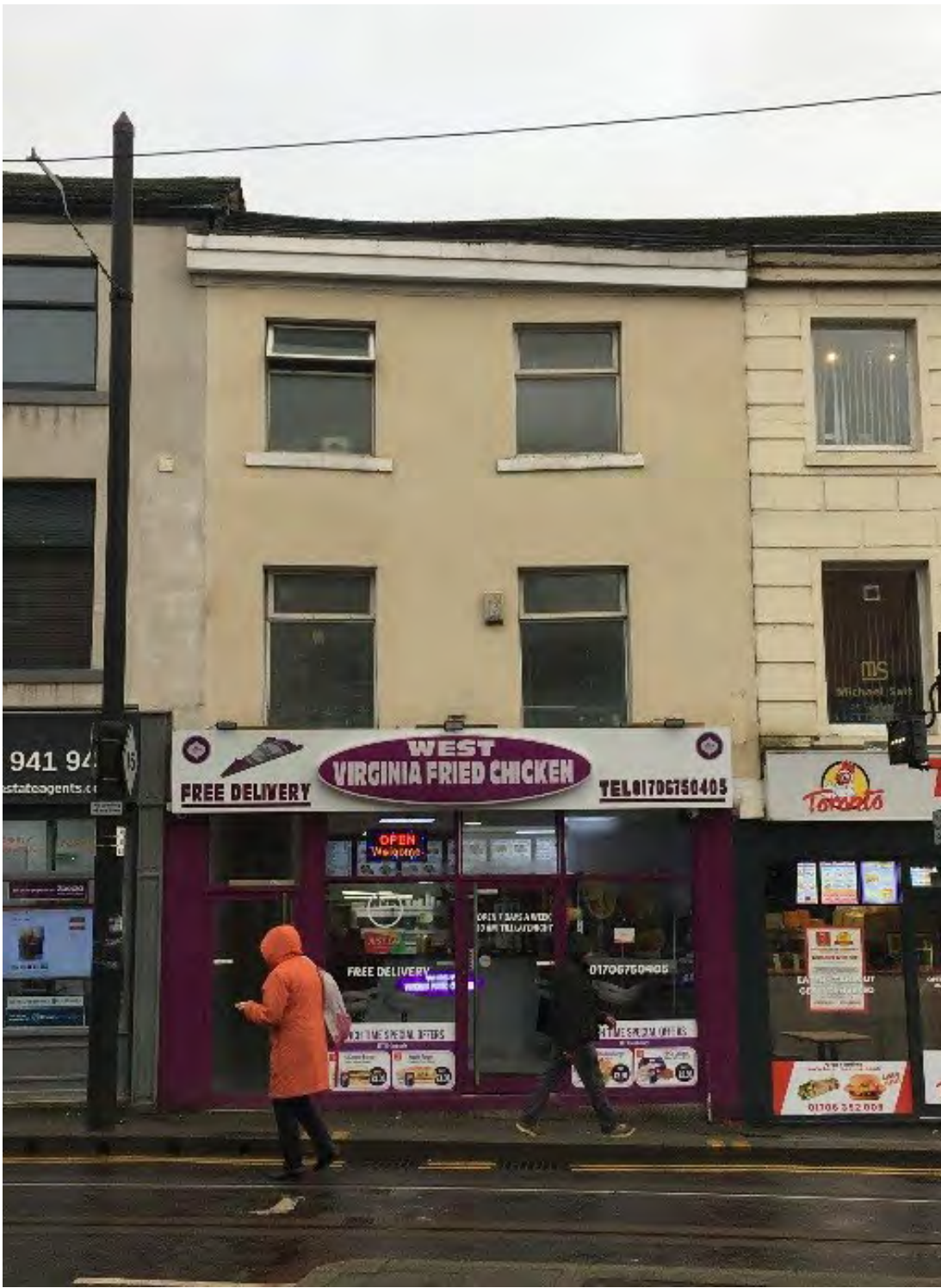
Figure 90: A current photograph of 4 Drake Street (Source: Purcell 2019).
