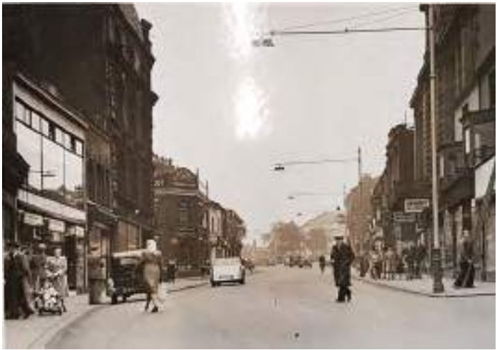
Figure 126: A 1955 photograph along Drake Street, showing the front elevation of 55 Drake Street with the earlier parapet and signage above the first floor to have been removed, but the shopfront appears to have retained its 19th century style timber-framed shopfront (Source: TR Dig Streets 513).
