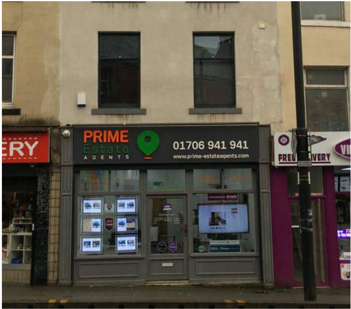
Figure 22: 6 Drake Street, showing the traditional style shopfront installed in 2018, utilising timber and good proportions and elements of a traditional shopfront, including: timber mullions separating the glass panes; a central door with a fanlight above; panelled stallrisers with cills; transom lights above the windows and doors; and decorative pilasters. (Source: Purcell 2019).
