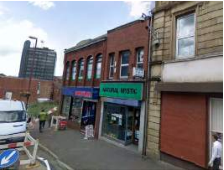
Figure 130: A 2008 photograph of Drake Street, showing 55 Drake Street with the existing shopfront, but with the previous 'Natural Mystic' signage (Source: Google 2008).
