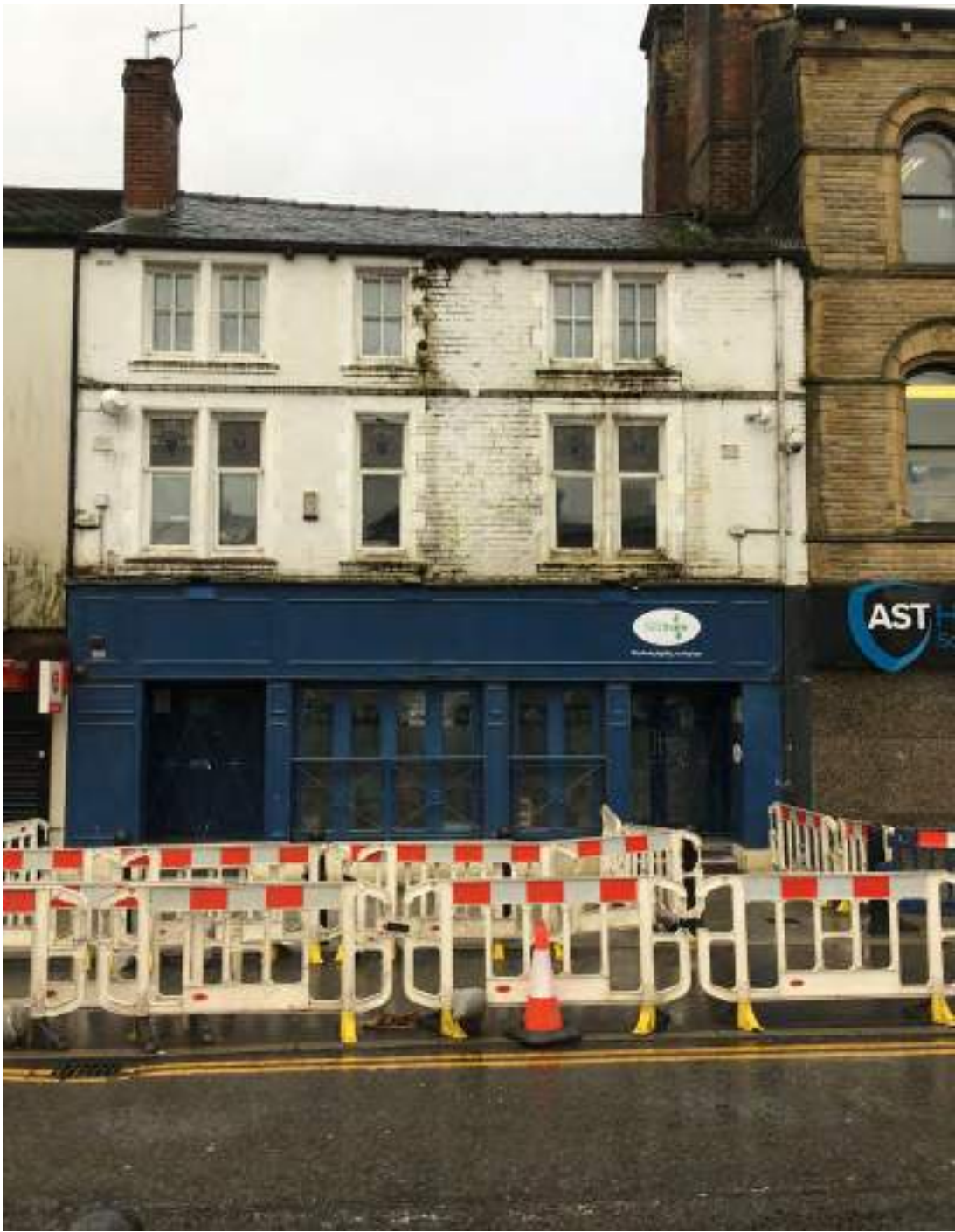
Figure 32: A current photograph of 8 South Parade (Source: Purcell 2019)
