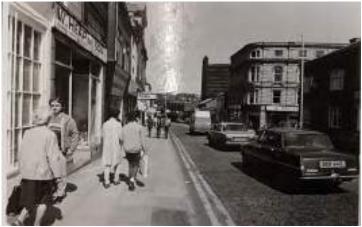
Figure 128: A c.1985-1987 photograph of Drake Street, showing 55 Drake Street on the right-hand side (Source: TR Dig Streets 2163).
