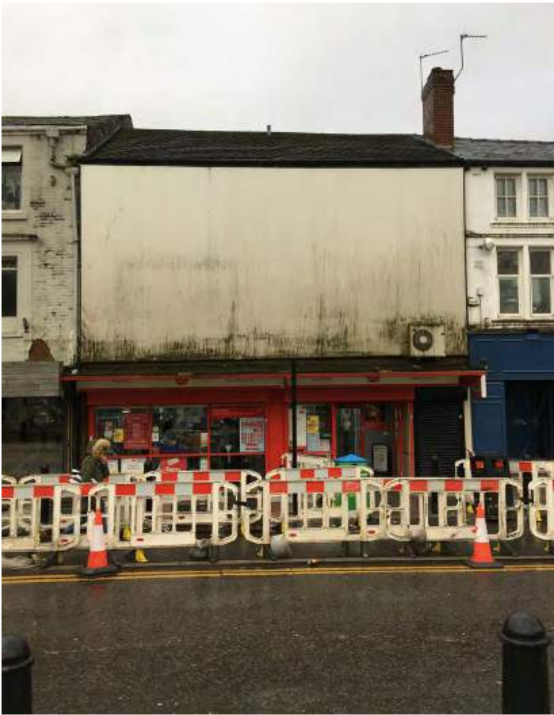
Figure 41: A current photograph of 9-10 South Parade (Source: Purcell 2019).
