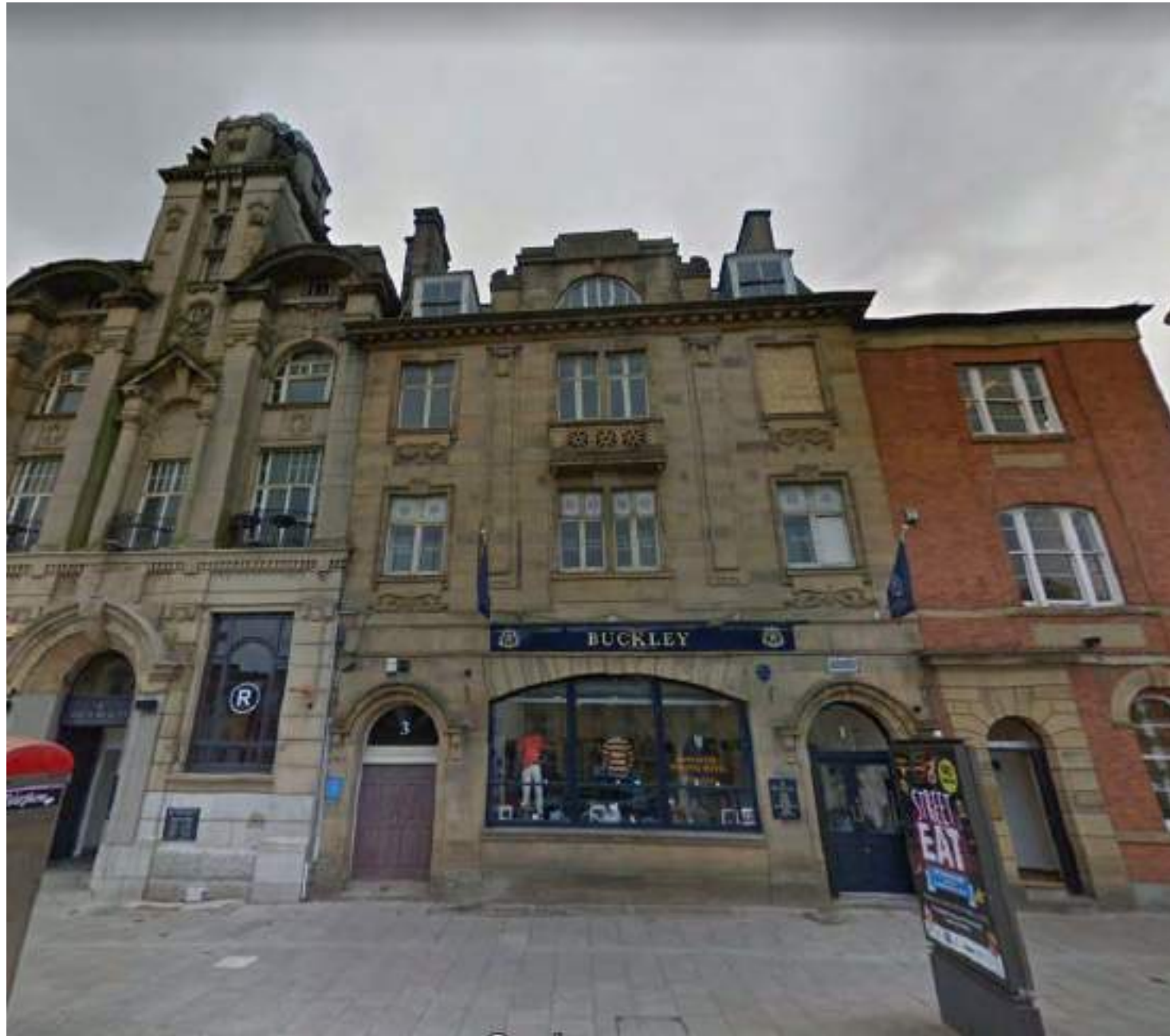
Figure 24: 1-5 South Parade, showing the retained early 20th century shopfronts (Source: Google 2019).
