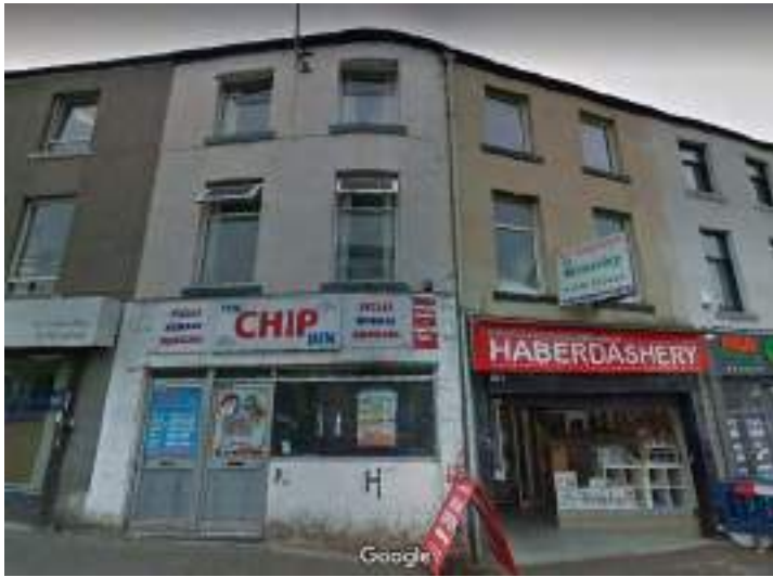
Figure 113: A 2018 Google Street View image of 10 Drake Street, showing the Chip Inn and its poorly painted and maintained c.1970s shopfront (Source: Google 2018).
