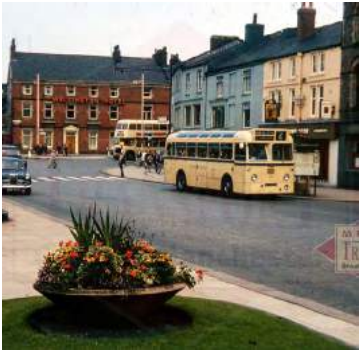
Figure 36: A 1960s photograph of South Parade, showing the shopfront at 8 South Parade replaced with a mid-20th century a frontage with a deep fascia and large windows, with the first and second floor elevation painted (Source: Museum of Transport Greater Manchester c.1960).
