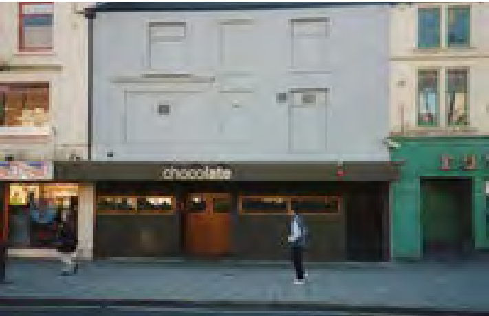
Figure 51: Photograph of 9-10 Drake Street in 2000, showing the infilled windows on the first and second floors, the cantilevered awning and the boxed-in shopfront, which were installed in 1993 (Source: Messenger 2000b).
