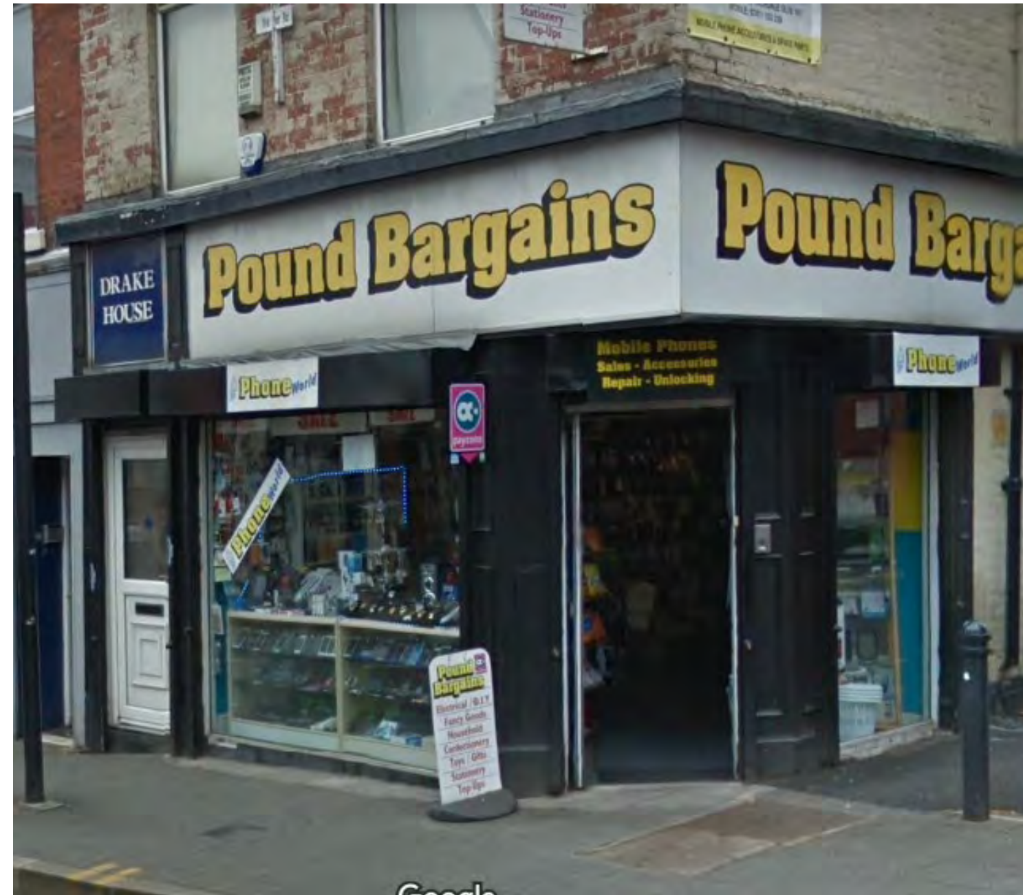
Figure 19: 21 Drake Street, showing timber panelled pilasters and a chamfered entrance as the only visible remains of a traditional shopfront, with unsympathetic deep fascia, projecting roller shutters and floor-length glass panes (Source: Google 2018).
