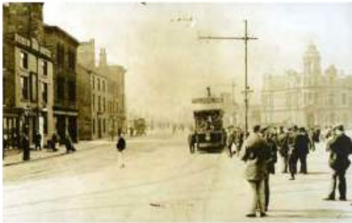
Figure 33: A historical photograph of 8 South Parade, c.1910, showing a three-storey two-bayed Georgian pub, known as the Robin Hood Hotel, with a central entrance on the ground floor front elevation with timber double-hung sashed windows on the ground to second floors, a timber parapet above the second floor and a central board fixed to the centre of the elevation (Source: Rochdale Local Studies c.1910a).
