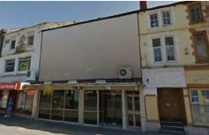
Figure 53: Photograph of 9-10 Drake Street in 2012, showing the re-painted canvas covering the first and second floors, a new cantilevered awning and a glazed aluminium-framed asymmetrical shopfront (Source: Google 2012).
