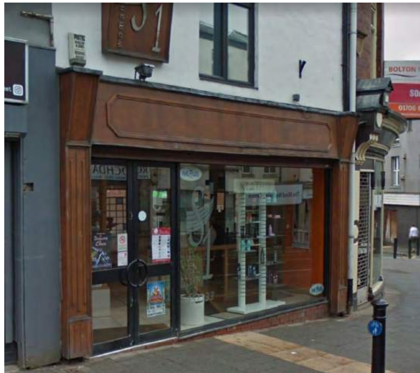
Figure 21: 16 Drake Street, showing a modern interpretation of a traditional shopfront, utilising timber fascia, plasters and corbels, inset with large unsympathetic aluminium-framed glass panes and door. (Source: Google 2018).
