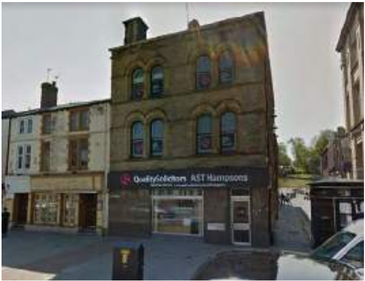
Figure 30: A 2012 Google Street View image of the front façade of 7 South Parade, showing the extant marble-clad shopfront and an earlier fascia signage (Source: Google 2012).
