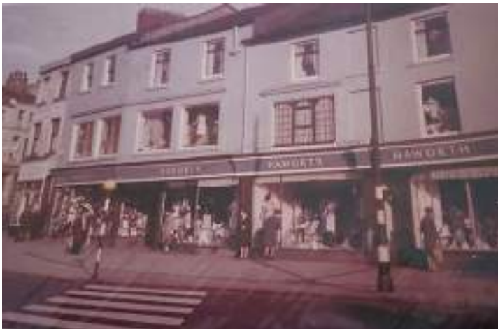
Figure 73: A c.1960 photograph of the front elevation at 9-12 South Parade, showing the refurbished shopfront at 12 South Parade (Source: 11-12 South Parade Archives c.1960).
