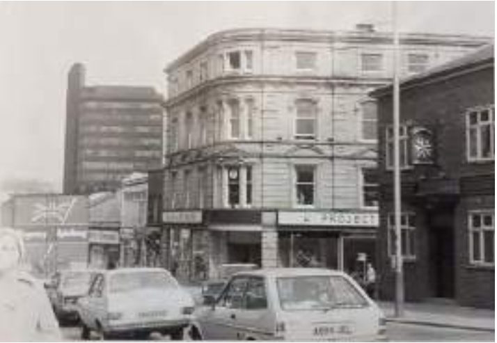
Figure 129: A 1980s photograph of Drake Street, showing 55 Drake Street on the right-hand side, with a large box awning installed above the shopfront (Source: TR Dig Streets 2159).
