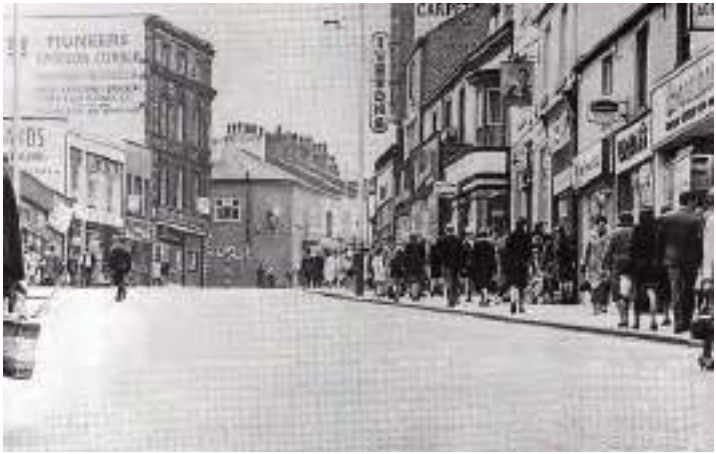
Figure 127: A 1965 photograph along Drake Street, showing the front elevation of 55 Drake Street showing shopfront to have been replaced with an unsympathetic shopfront (Source: Rochdale Local Studies).
