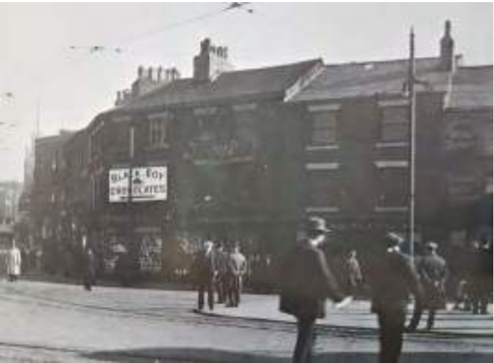
Figure 45: A c.1920s photograph of the corner of Drake Street and South Parade, showing only the eastern section of the front elevation of 9-10 South Parade. The windows on the first and second floors are eight-over-eight timber double-hung sashed windows, adjacent to a timber advertising board, but the ground floor shopfront is difficult to make out other than the glazing on the windows and the eastern door (Source: TR Dig Streets 501).
