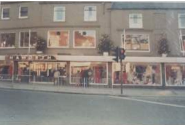
Figure 65: A c.1982 photograph of the front elevation at 9-12 South Parade, showing 11 South Parade to have to be reconfigured with the continuous awning along the front façade, as well as the alterations of the entrances and introduction of very large aluminium-framed windows (Source: 11-12 South Parade Archives c.1982).
