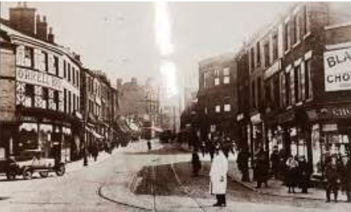
Figure 92: A c.1920s photograph of Drake Street from South Parade, showing the front elevation of 4 Drake Street to comprise a rendered first and second storey with decorated Art Deco surrounds around the originally Georgian windows and a mid-19th century style timber-framed shopfront with a wide fascia, narrow glass panes and a small parapet and balustrading above a projecting cornice (Source: TR Dig Streets 2167).
