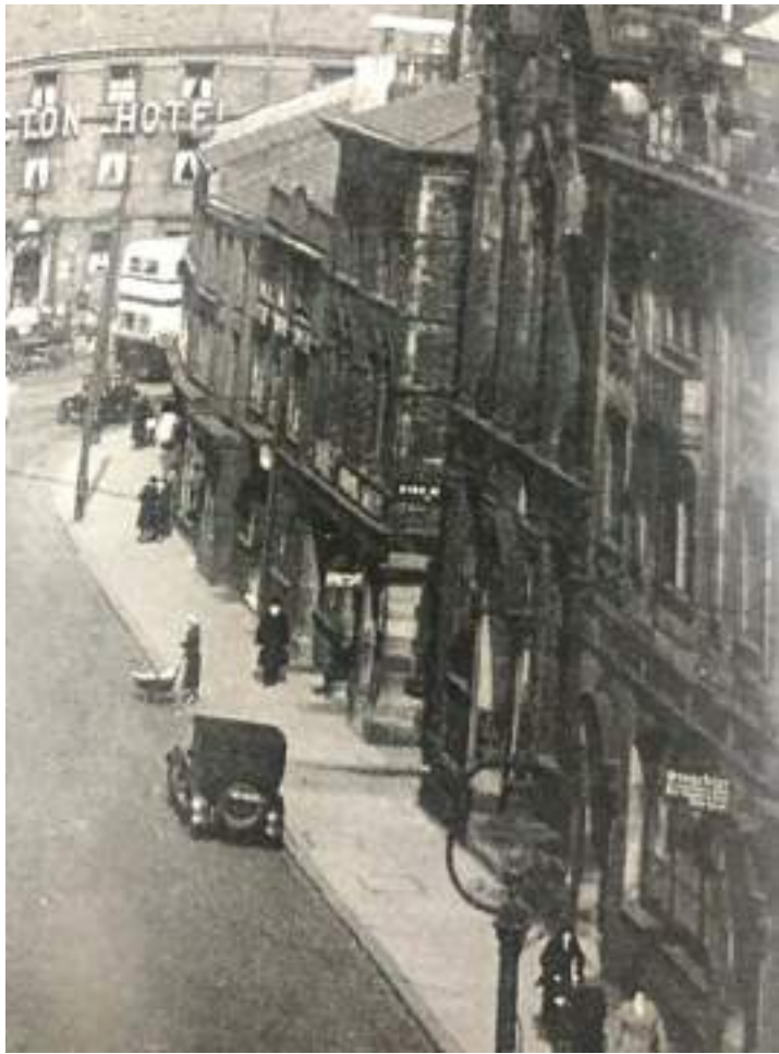
Figure 27: A historical photograph of 7 South Parade, c.1914, showing the earlier stone-faced frontage of the ground floor front elevation (Source: Rochdale Local Studies).
