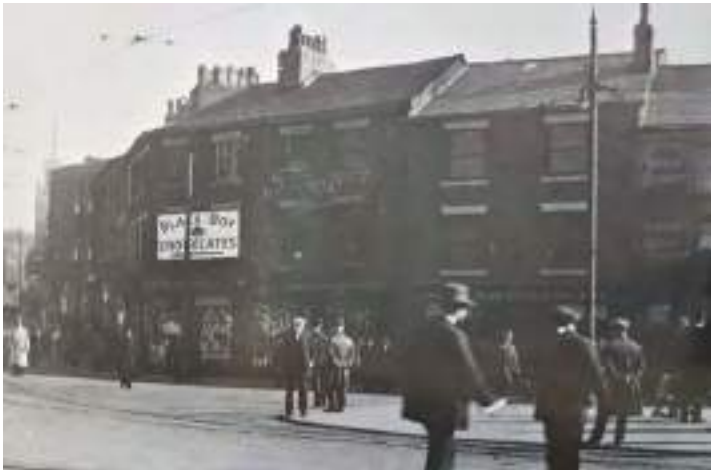
Figure 69: A c.1920s photograph of the corner of Drake Street and South Parade, showing the front elevation of 12 South Parade to comprise a two-bay three storey building exposed brick with single-paned double-sashed timber sashed windows on the first and second floors. The shopfront appears to be a late 19th century style timber-framed shopfront with a thin fascia, used by Haworth, a clothing store (Source: TR Dig Streets 501).
