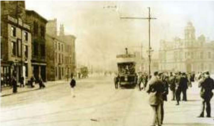
Figure 43: A historical photograph of a small section of the shopfront at 9 South Parade, dated to c.1910, showing a timber fascia and cornice above timber-framed windows and a timber pilaster on the ground floor (Source: Rochdale Local Studies c.1910a).
