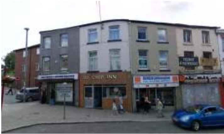
Figure 112: A 2008 Google Street View image of 6 to 12 Drake Street, showing the Chip Inn and its unsympathetic c.1970s shopfront at 10 Drake Street (Source: Google 2008).
