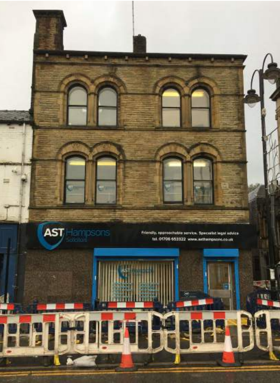
Figure 25: A current photograph of 7 South Parade (Source: Purcell 2019).
