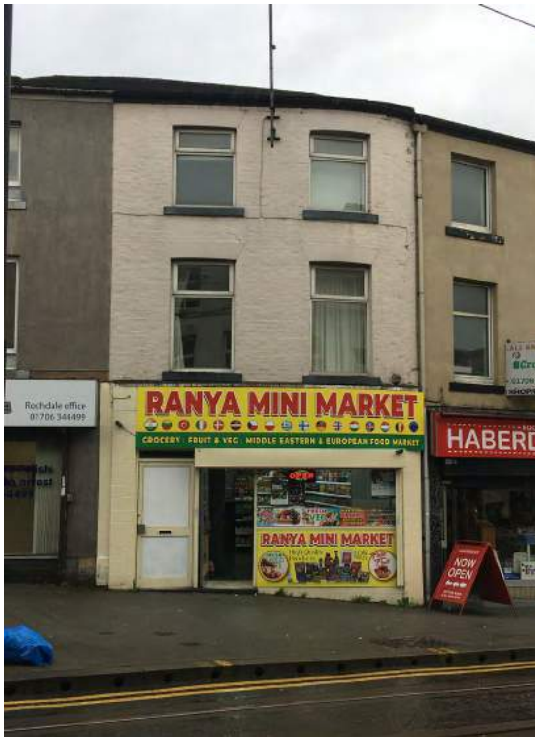
Figure 107: A current photograph of 10 Drake Street (Source: Purcell 2019).
