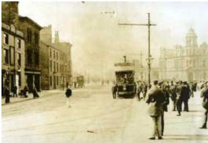
Figure 25: A historical photograph of 7 South Parade, c.1910, showing a three-storey two-bayed stone-faced building with double-windows on the first to second floors, a deep cornice above and what appears to be a timber-framed fascia and cornice above stone pilasters (Source: Rochdale Local Studies c.1910a).
