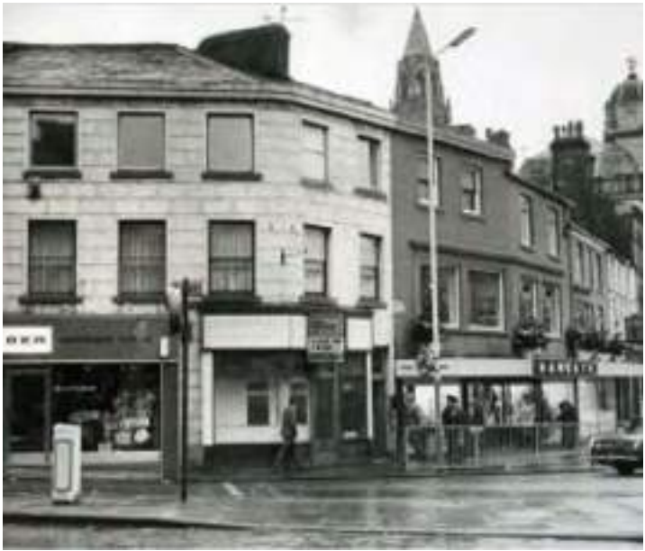
Figure 37: A c.1970s photograph of Drake Street and South Parade, showing 8 South Parade with a late-20th century shopfront, c.1930s windows and a hanging sign for the Robin Hood Public House (Source: Rochdale Local Studies c.1970a).
