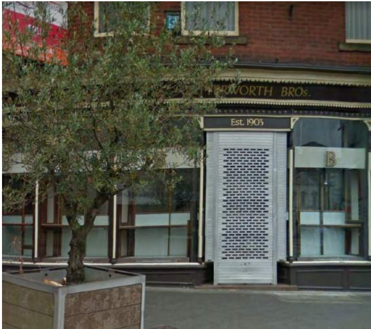
Figure 18: 14 Drake Street, showing the retained appearance of the historic 1903 shopfront of Butterworth Bros., with its decorative angled fascia and cornice above, decorative pilasters with plinth, capital, corbel and letterbox, timber panelled stallrisers, decorative timber mullions between glass pane and hand-painted signage directly onto the fascia (Source: Google 2018).
