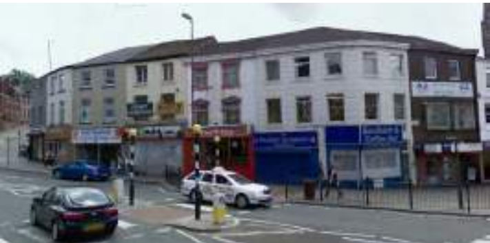
Figure 89: A 2008 Google Street View image of 13 South Parade/2 Drake Street through to 12 Drake Street, showing the Sandwich and Coffee Bar and its unsympathetic shopfront at 13 South Parade/2 Drake Street, including partially perforated roller shutters (Source: Google 2008).
