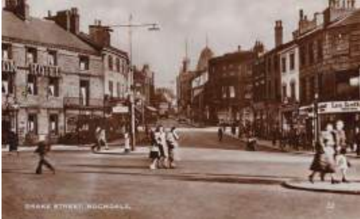
Figure 85: A mid-1930s photograph of Drake Street, showing the front elevations of 13 South Parade and 2 Drake Street to have been rendered with a deeply scoured stone ashlar pattern continuing across both properties, likely undertaken in the 1920s or 1930s, indicating their connection from the first half of the 20th century. The ground floor shops were used by Lea-Scott Opticians and what appears to be O. Loyts, with the first floor and second floor used by J.W. Dutton and a hairdressers, respectively (Source: Ashworth 2018).
