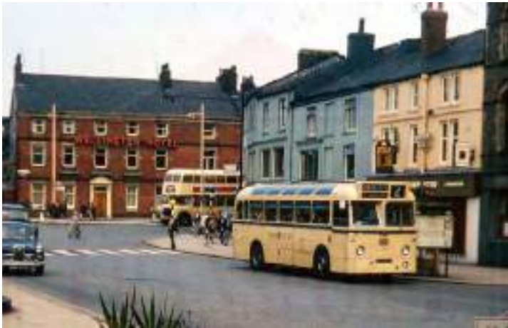
Figure 74: A 1960s photograph of South Parade, showing the front elevation at 12 South Parade with its c.1920s or 1930s large windows on the first floor (Source: Museum of Transport Greater Manchester c.1960).
