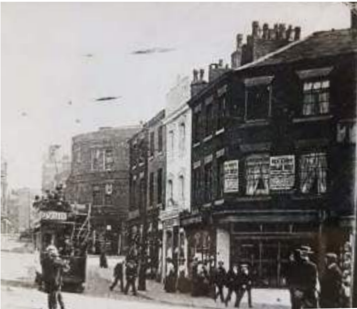
Figure 91: A c.1910 photograph of Drake Street from South Parade, showing the front elevation of 4 Drake Street to comprise a rendered façade with pedimented window surrounds on the first and second floors, a decorative parapet above the second floor, and a 19th shop frontage with a timber fascia and cornice, an ornamental pediment above the cornice, a recessed doorway and timber-framed glazing (Source: TR Dig Streets 510).
