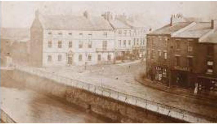
Figure 68: The earliest photograph obtained of the property, dating to c.1855, showing the corner of Drake Street and South Parade, showing the front elevation of 12 South Parade to comprise a two-bay three-storey Georgian terraced building with exposed brickwork and timber framed windows, with a ground floor mid-19th century symmetrical timber-framed shopfront on the ground floor. The windows on the first floor were likely extended in length in the Victorian period to provide more light in the room (Source: TR Dig Streets 545).
