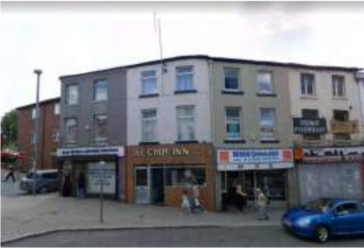
Figure 106: A 2008 Google Street View image of 6 to 12 Drake Street, showing the Rochdale Communications and its unsympathetic c.1970s shopfront and 1980s tiles at 8 Drake Street (Source: Google 2008).
