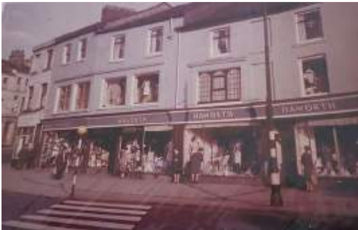
Figure 47: A c.1960 photograph of the front elevation at 9-12 South Parade, showing 9-10 South Parade to have infilled windows of the central bay on the first and second floors, as well as the c.1920s/early 1930s large window in the eastern bay of the first floor and the c.1940s timber-framed windows with hinged transoms (Source: 11-12 South Parade Archives c.1960).
