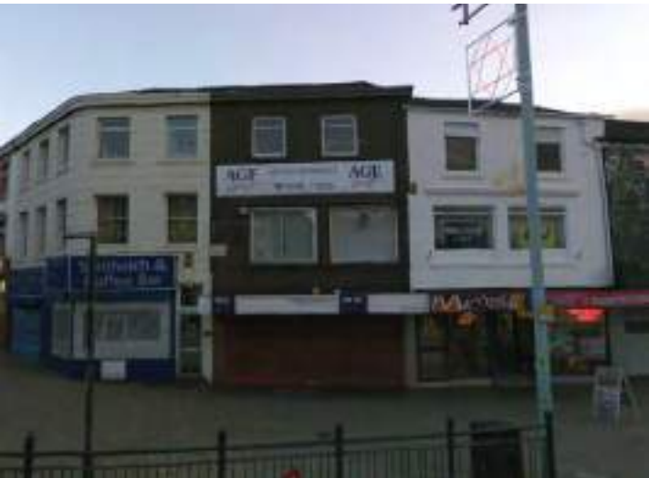
Figure 79: A 2008 photograph of 11 South Parade used as a fried chicken restaurant on the ground floor with a 1984 shopfront (Source: Google 2008).
