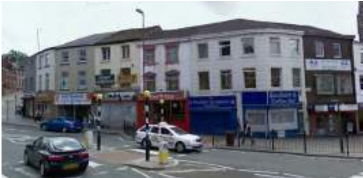
Figure 97: A 2008 Google Street View image of 13 South Parade/2 Drake Street through to 12 Drake Street, showing the Pizza King and its unsympathetic shopfront at 4 Drake Street, installed in 1994 (Source: Google 2008).
