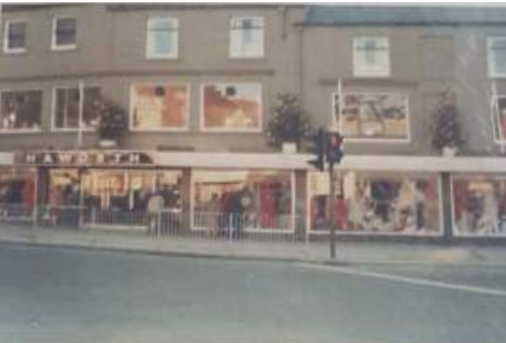
Figure 78: A c.1982 photograph of the front elevation at 9-12 South Parade, showing 12 South Parade to have to be reconfigured with the continuous awning along the front façade, as well as the alterations of the entrances and introduction of very large aluminium-framed windows (Source: 11-12 South Parade Archives c.1982).
