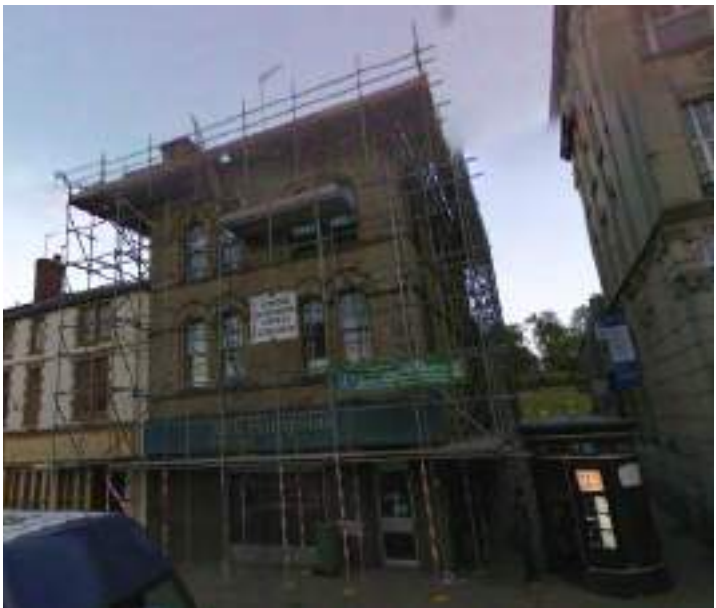
Figure 29: A 2008 Google Street View image of the front façade of 7 South Parade, showing the extant marble-clad shopfront and the earlier fascia signage (Source: Google 2008).
