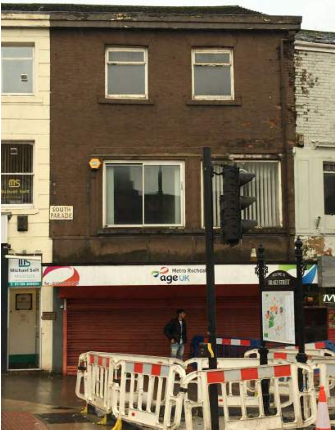
Figure 67: A current photograph of 12 South Parade (Source: Purcell 2019).
