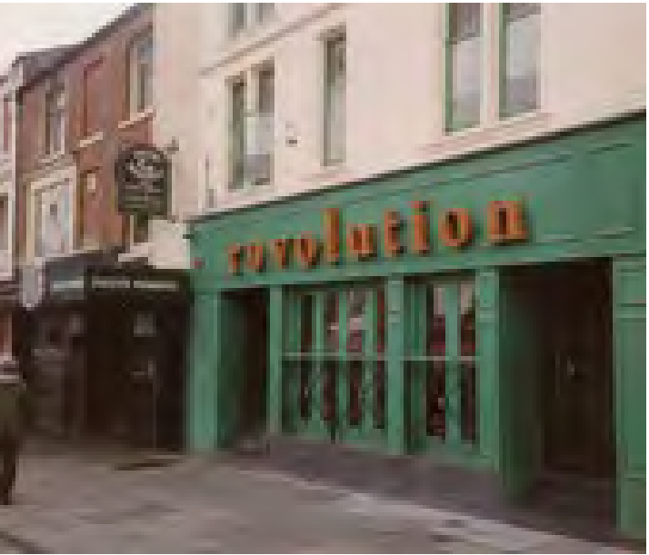
Figure 39: A 2000 photograph of South Parade, showing 8 South Parade with the c.1930s first and second floor windows, but with replaced glazing in the lower panes, as well as the existing timber-panelled shopfront with large recessed doors and a deep fascia (Source: Messenger 2000a).
