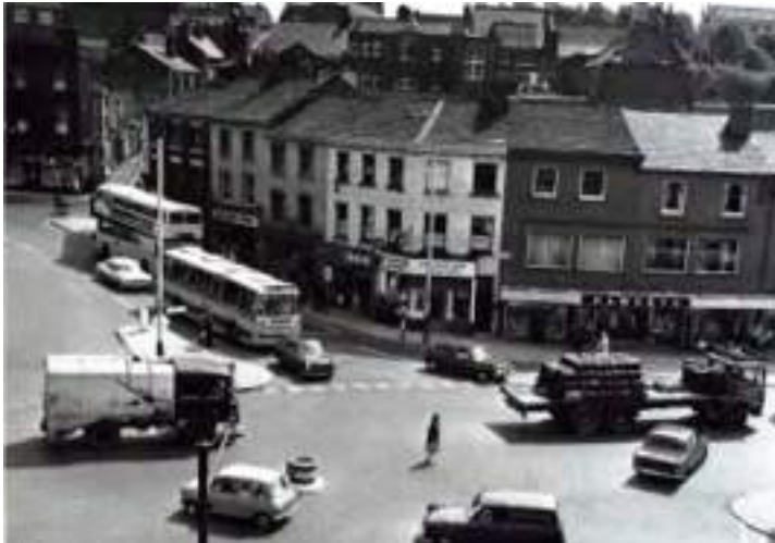
Figure 95: A c.1966/67 photograph of Drake Street and South Parade. The rendered front elevation and Art Deco window surrounds of 4 Drake Street appears to have been retained, as well as the 19th century shopfront (Source: Rochdale Local Studies 1966/67).
