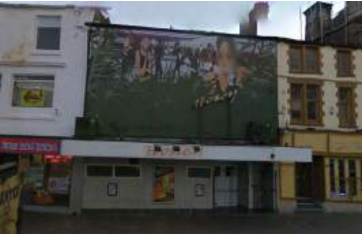
Figure 52: Photograph of 9-10 Drake Street in 2008, showing the painted canvas covering the first and second floors, the cantilevered awning and the tiled boxed-in shopfront (Source: Google 2008).
