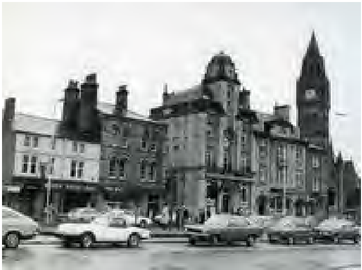
Figure 38: A c.1970s photograph of South Parade, showing 8 South Parade with the c.1930s windows and an asymmetrical shopfront with large recessed doors and a deep fascia (Source: Rochdale Local Studies c.1970b).
