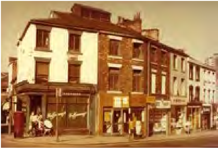
Figure 96: Photograph of 2-12 Drake Street, showing 4 Drake Street in the background (Source: Anstess 1981a).
