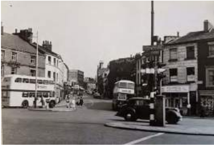
Figure 102: A c.1965 photograph of Drake Street, showing the earlier shopfront at 8 Drake Street to have been replaced with a mid-20th century symmetrical frontage with a tall, deep inclined fascia. The first and second floor elevations still comprised exposed brickwork at this time (Source: TR Dig Streets 114).
