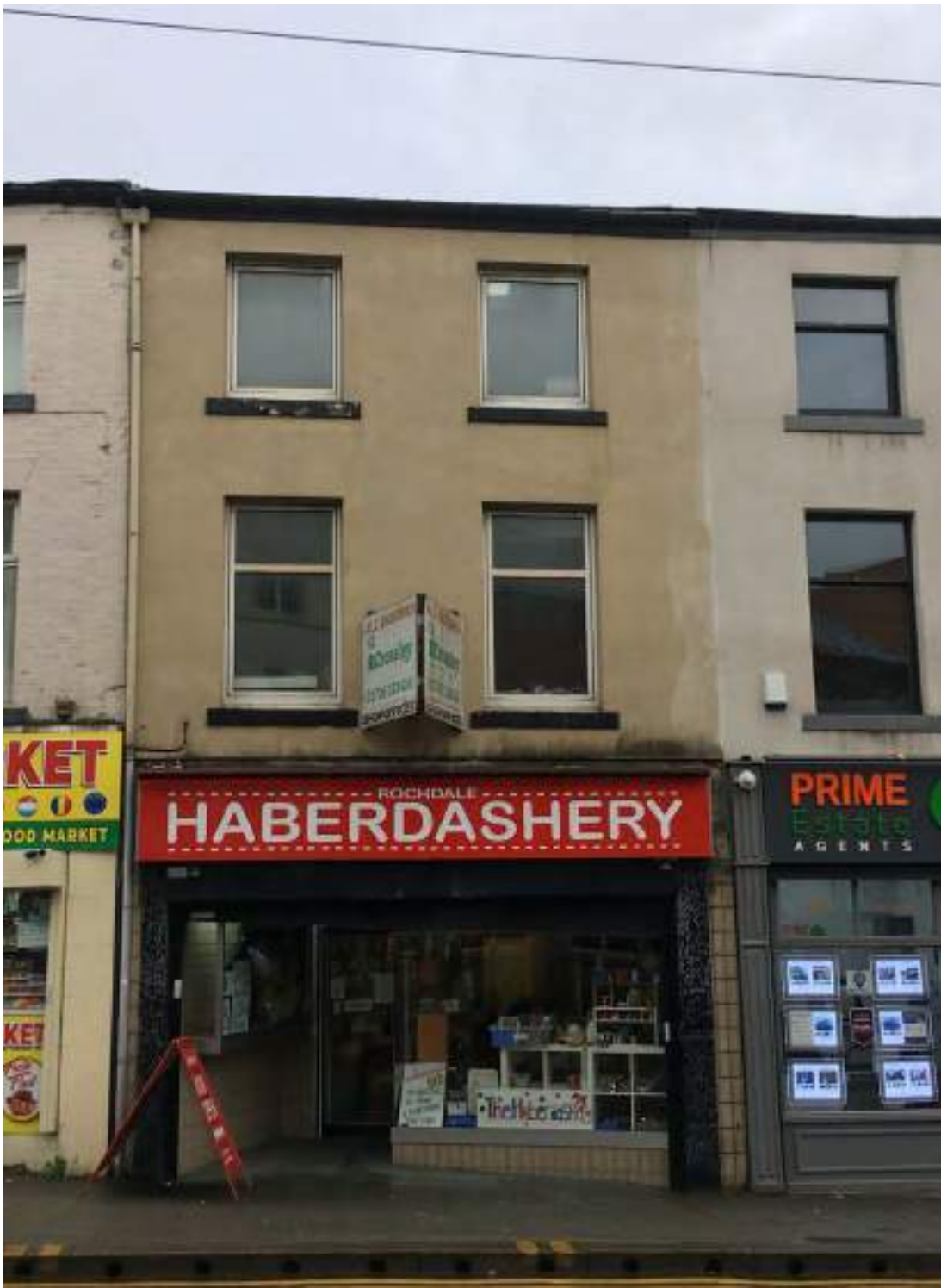
Figure 98: A current photograph of 8 Drake Street (Source: Purcell 2019).
