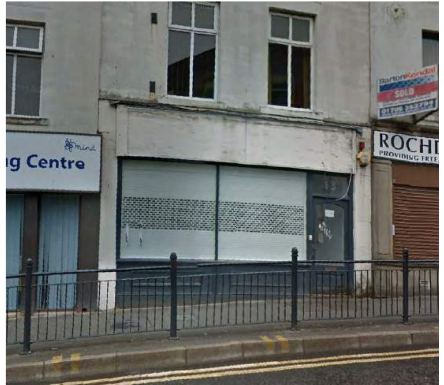
Figure 17: 13 Drake Street, showing the slightly recessed timber panelled stallriser, timber mullion separating two glass panes, fanlight above the door and timber door of the 19th century shopfront, though a number of elements appear to have been reproduced. However, the fascia is too deep and in poor condition and there are no pilasters (Source: Google 2018).
