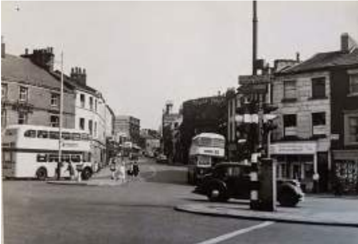
Figure 94: A c.1965 photograph of Drake Street, showing the rendered front elevation and Art Deco window surrounds of 4 Drake Street to have been retained, as well as the 19th century shopfront (Source: TR Dig Streets 114).
