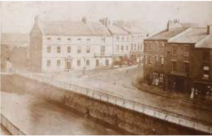
Figure 55: The earliest photograph obtained of the property, dating to c.1855, showing the corner of Drake Street and South Parade, showing the front elevation of 11 South Parade to comprise a two-bay three-storey Georgian terraced building with exposed brickwork and eight-over-eight paned vertically sliding timber sashed windows, with a symmetrical timber-framed shopfront on the ground floor (Source: TR Dig Streets 545).
