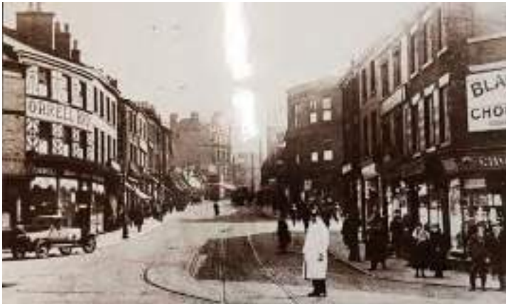
Figure 83: A c.1920s photograph of Drake Street from South Parade, showing the front elevation of 13 South Parade and 2 Drake Street to comprise exposed brick with timber sashed windows and advertising boards fixed next to and in front of windows. The shopfronts appear to be 19th century style timber-framed shopfronts with diagonal fascia at 13 South Parade and an early 20th century style box fascia at 2 Drake Street (Source: TR Dig Streets 2167).
