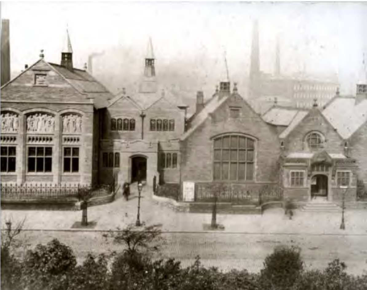
Fig.10 Above: Photograph Showing First & Second Phases
