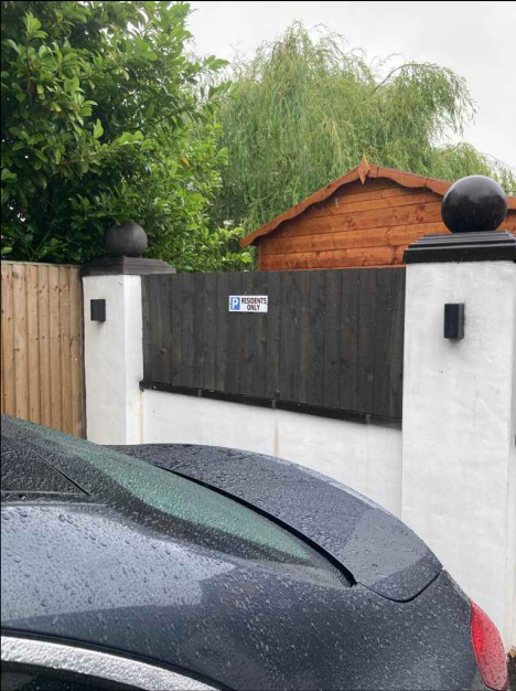
green dotted line indicates extents of block rendered wall with timber infill panels
