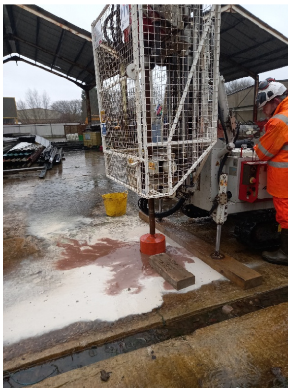
Photograph 2 — BH01; Concrete coring
