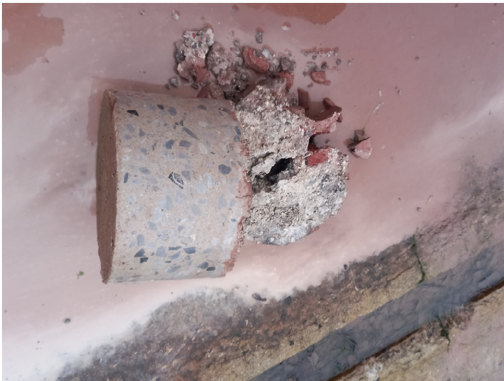
Photograph 3 — BH01; Concrete core
