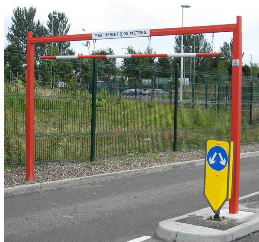
Example images of typical automatic entrance gate and height restrictor to proposed car park entrance point 3 (Preliminary design only - subject to amendment by manufacturer)
