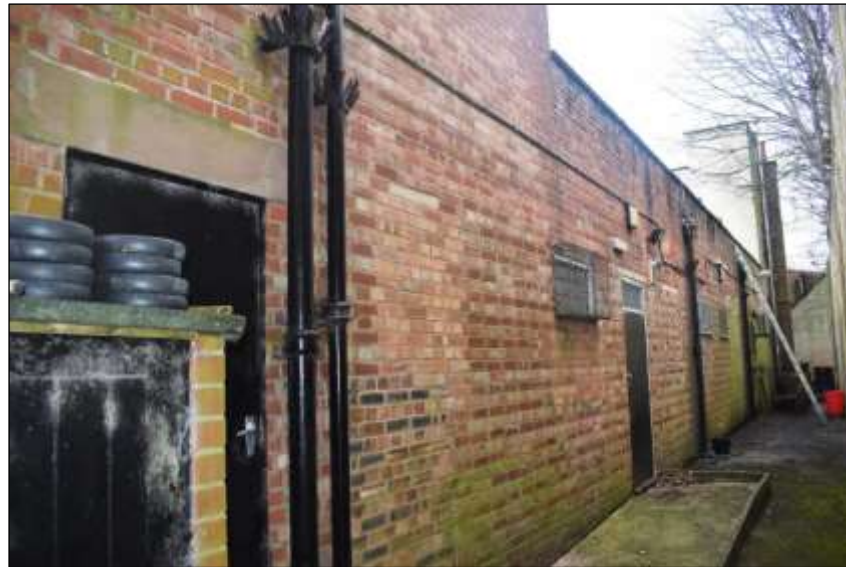
Photo 5: 18 Sadler Street rear elevation, looking west
