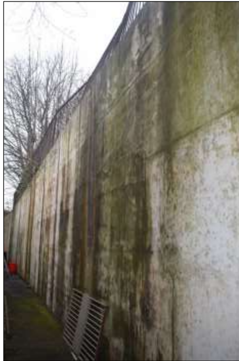
Photo 7: Retaining wall along north of 18 Sadler Street plot
