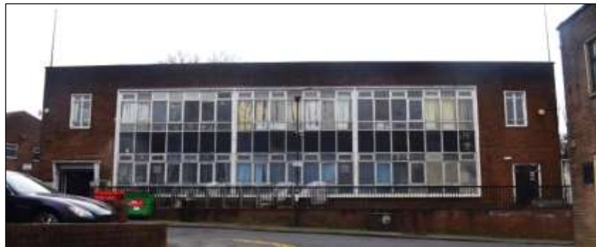
Photo 1: 18 Sadler Street, facade, looking north-west
