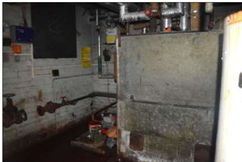
Photo 6: 18 Sadler Street, basement boiler / generator room
