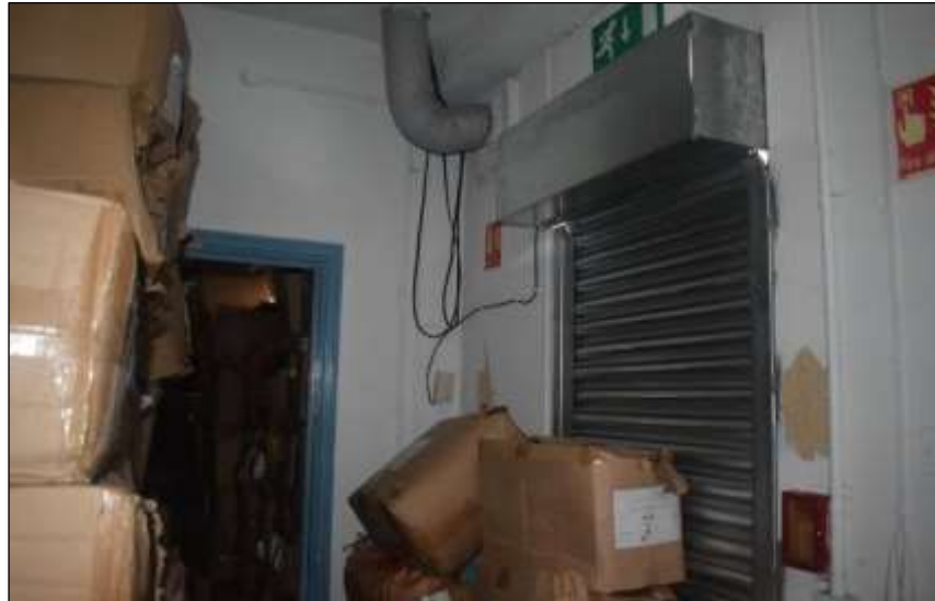
Photo 9: 18 Sadler Street, rear of ground floor, general view
