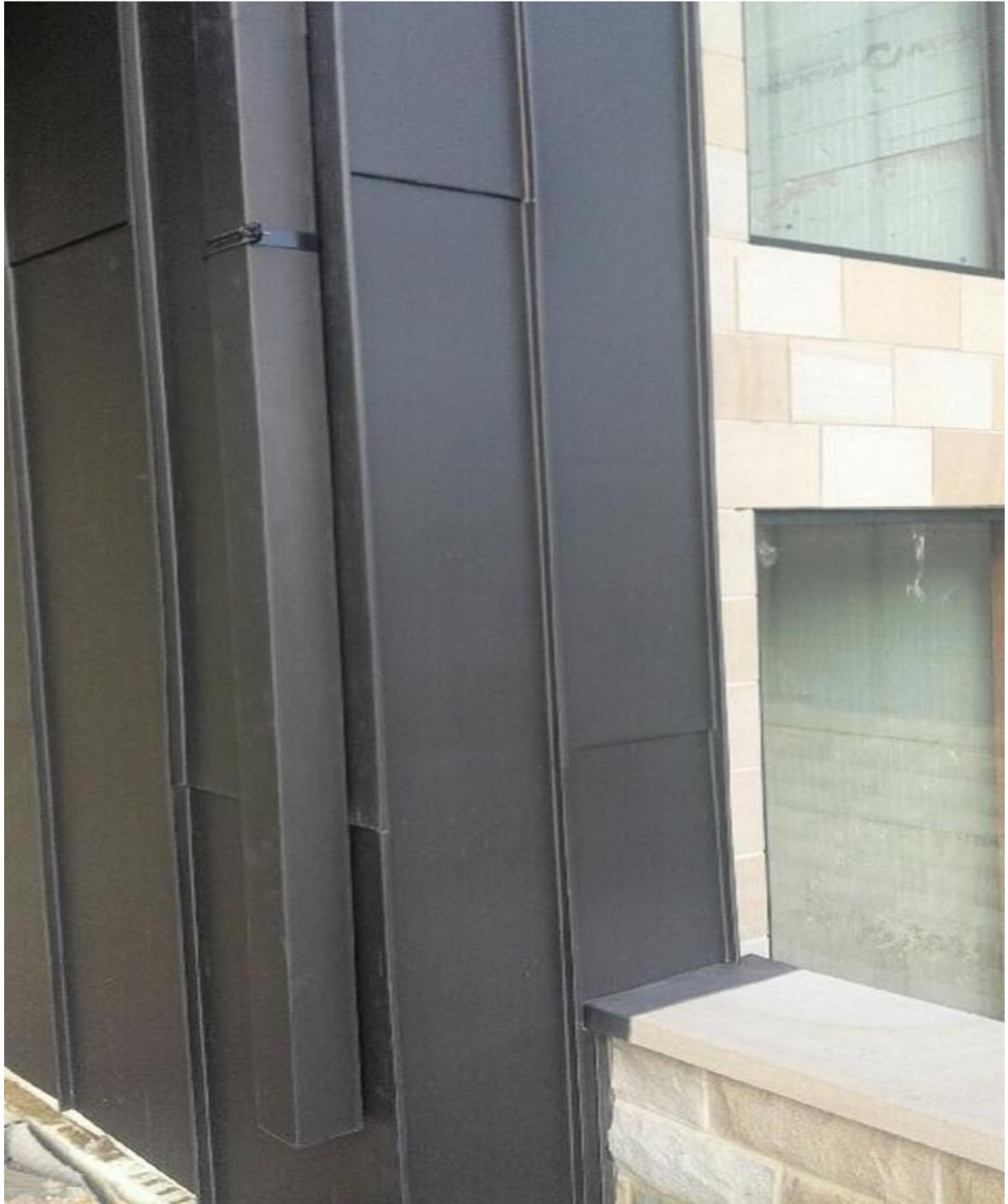
Photo of Zinc Cladding Wall Finish for Mill House Farm
