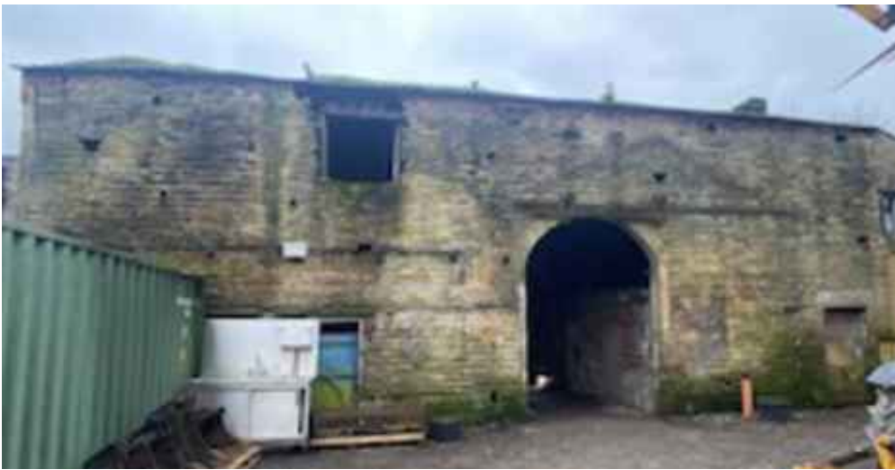
Existing Rear Elevation (photo)
