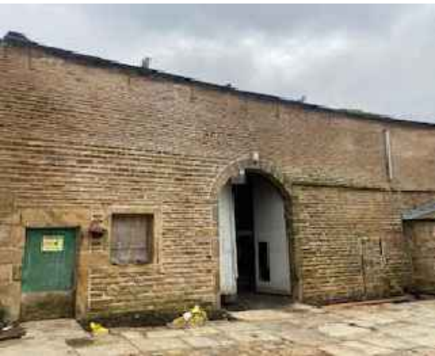
Existing Front Elevation (photo)
