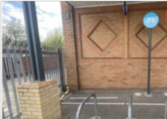
PHOTOGRAPH OF EXISTING ELEVATION A
