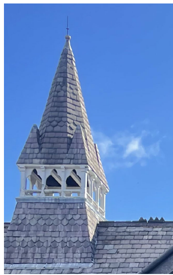
Cupola tiling intact
