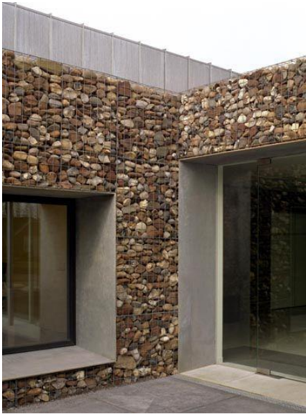
deep reveals to super-insulated walls
