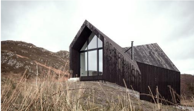
charred timber cladding
