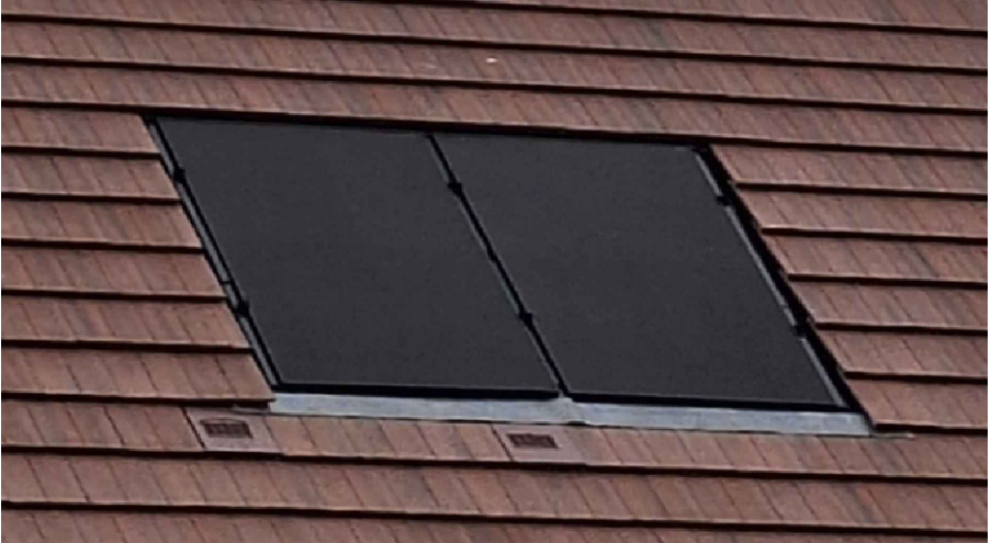
As built photo of PV panels
