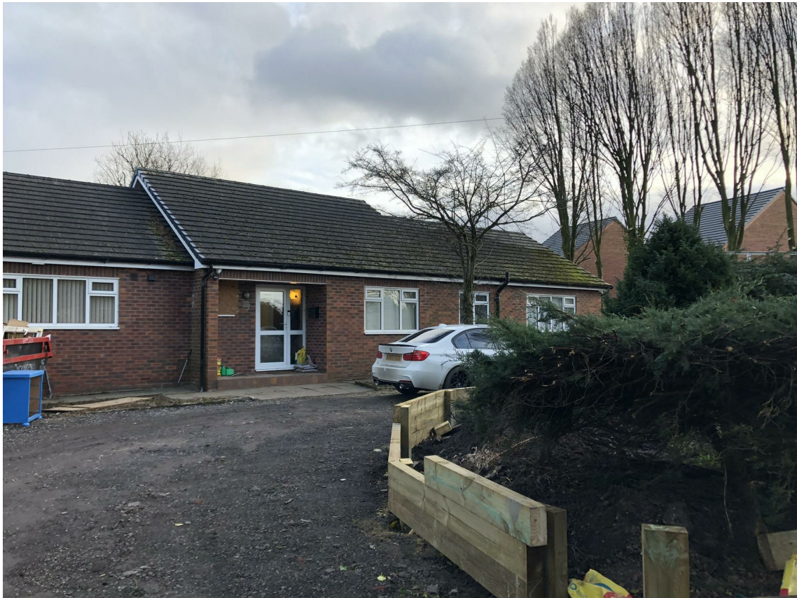
EXISTING FRONT ELEVATION - VIEW 1
