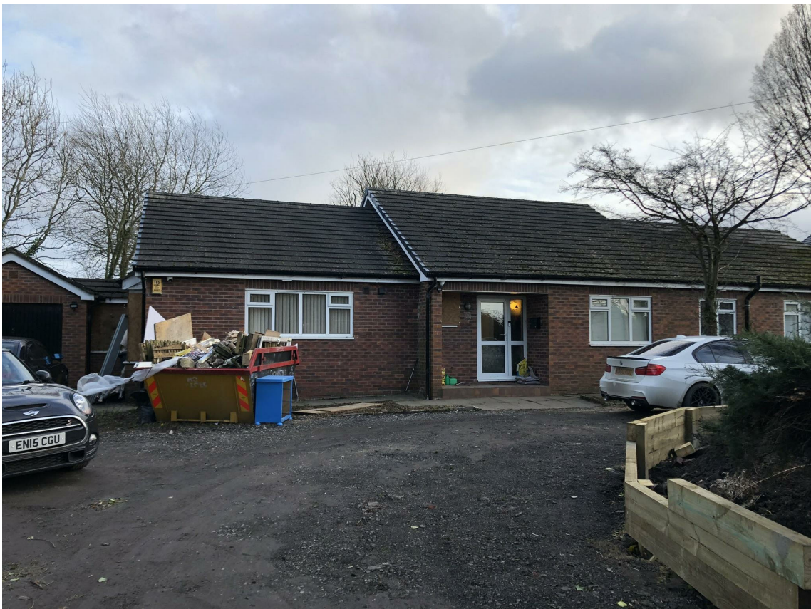
EXISTING FRONT ELEVATION - VIEW 2
