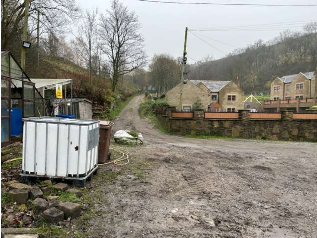
Plate 5 - View from subject site with access passing to east of Carp View
