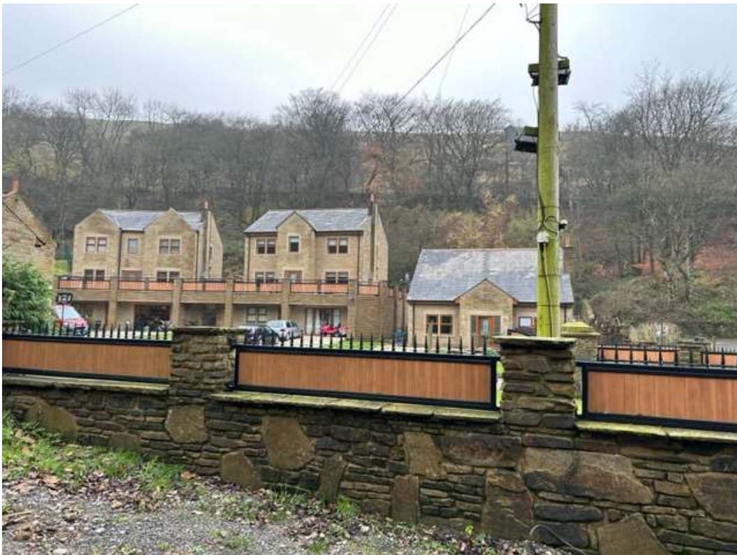
Plate 6 – View from access to east boundary of Carp View
