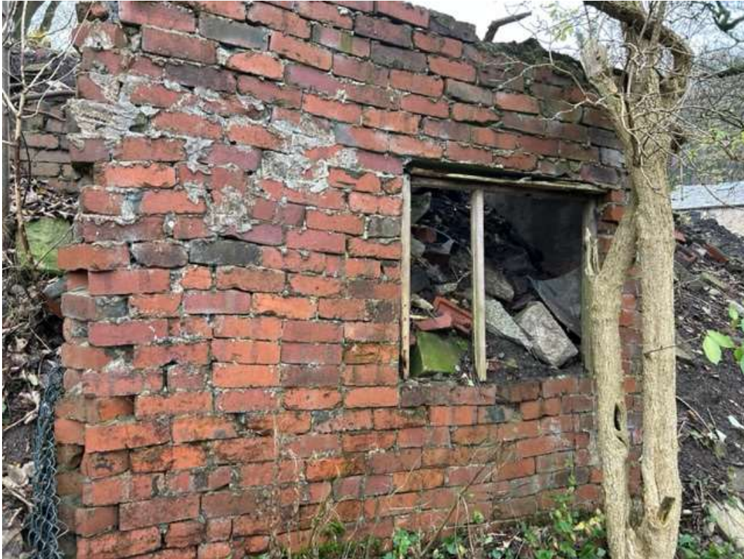
Plate 17 – Brick structure from Mill use located at north boundary
