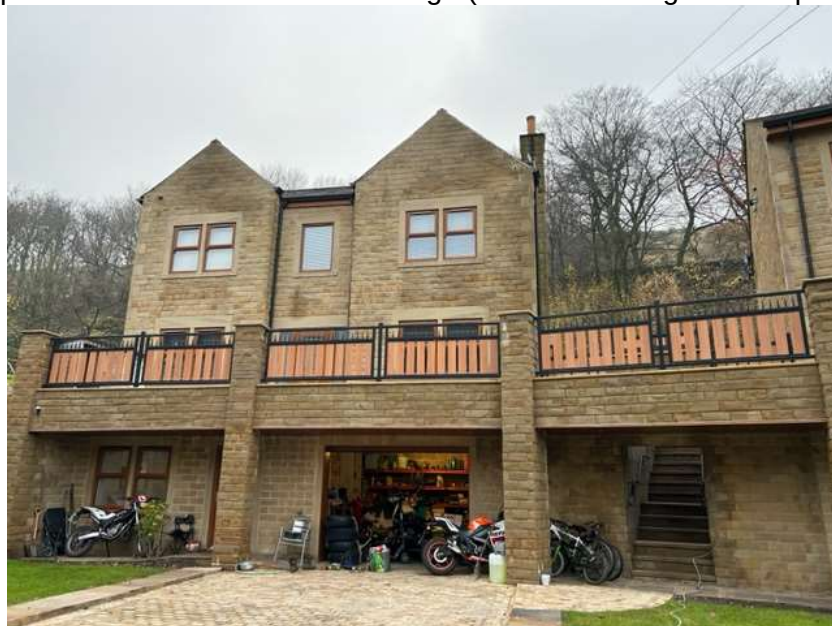
Image 5 – Three storey build at Carp View
