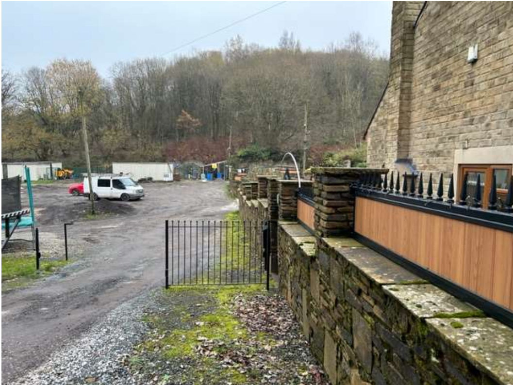
Plate 11 – View of site from access adjacent to 1 Carp View
