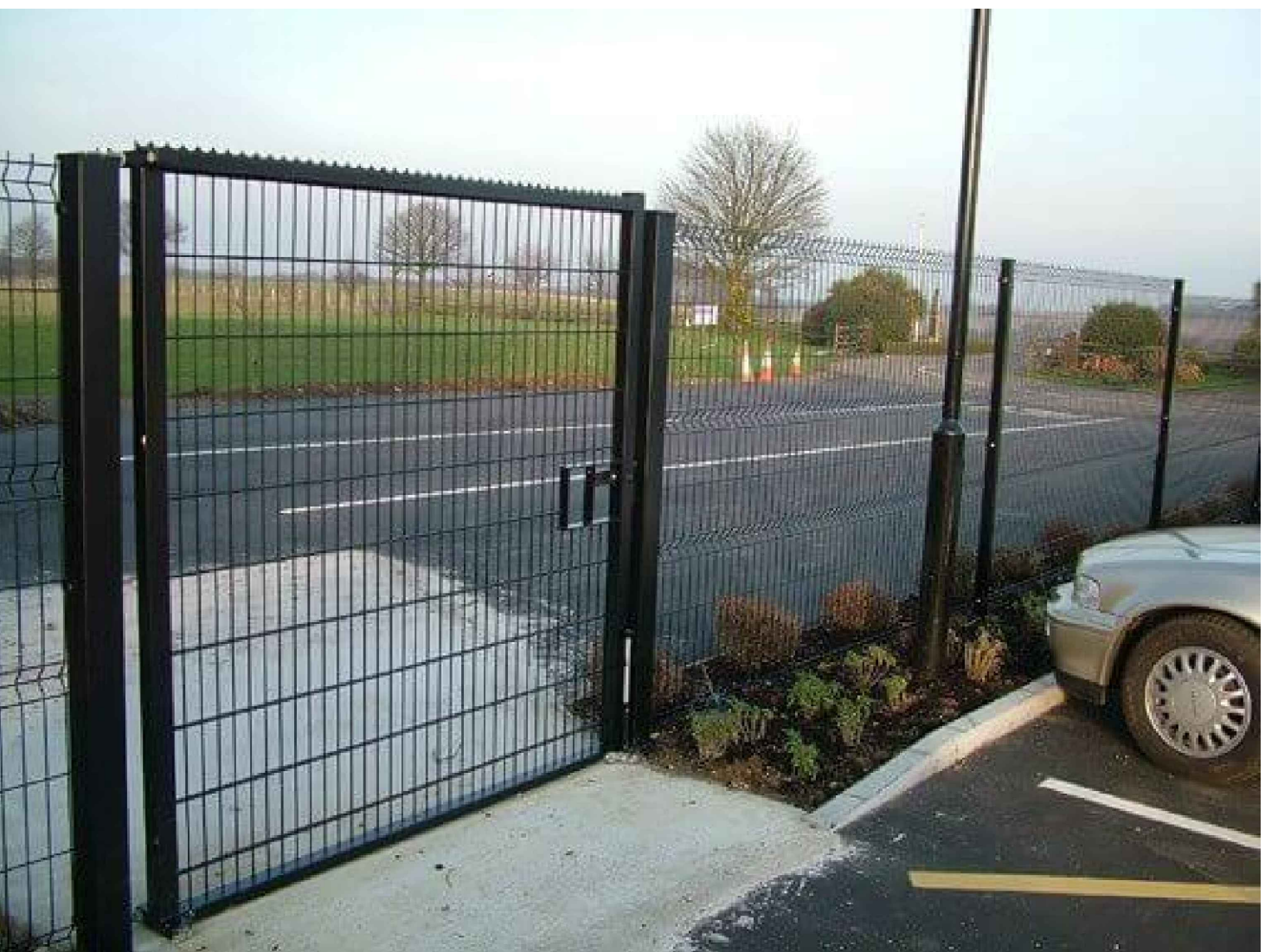
TYPICAL PHOTO OF FENCE & GATE
