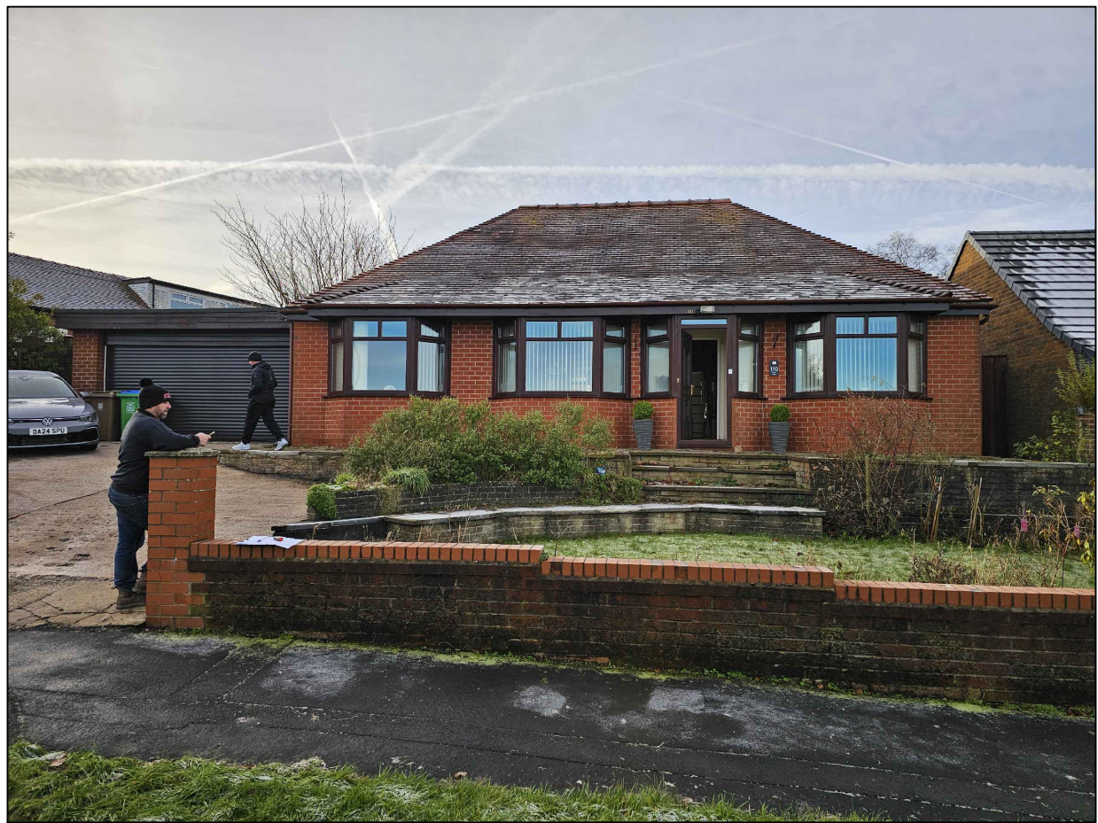
Site Photo-Existing Front Elevation
