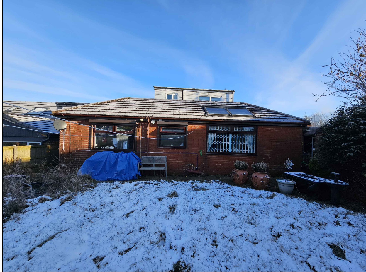
Site Photo-Existing Rear Elevation
