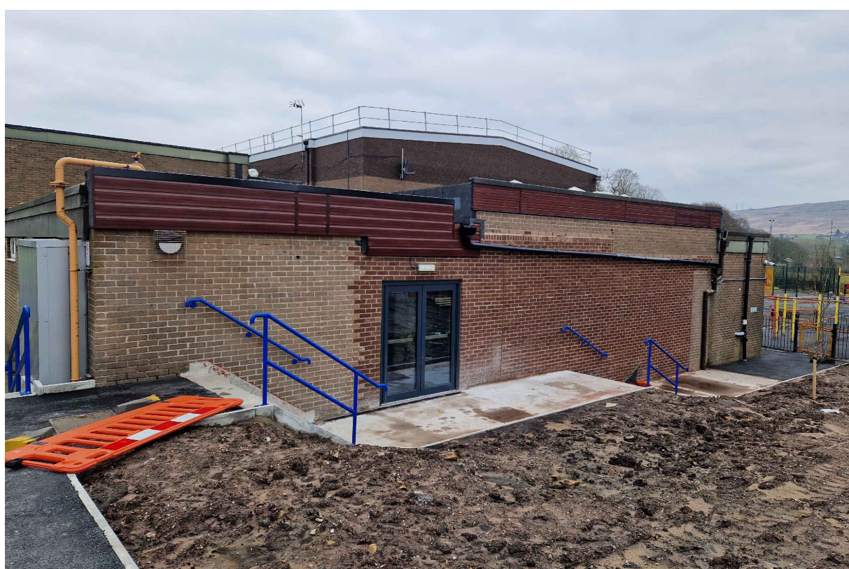
PHOTO OF EXISTING SOUTH ELEVATION - NTS
