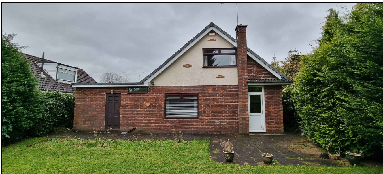
Site Photo-Existing Rear Elevation (N.T.S)
