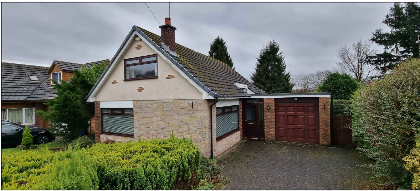
Site Photo-Existing Front Elevation (N.T.S)
