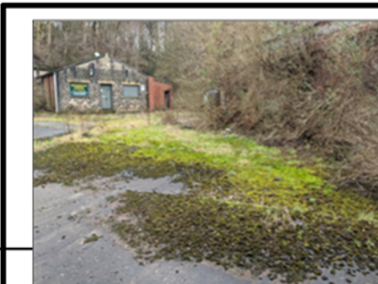
SITE 2 - EXISTING EXTERIOR BUILDING 2
