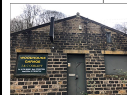
SITE 2 - EXISTING EXTERIOR BUILDING 2
