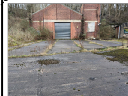
SITE 2 - EXISTING EXTERIOR BUILDING 1
