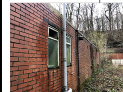
SITE 2 - EXISTING EXTERIOR BUILDING 2
