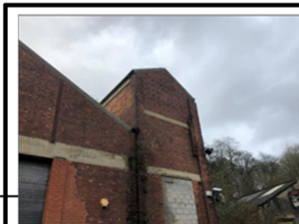
SITE 2 - EXISTING EXTERIOR BUILDING 1
