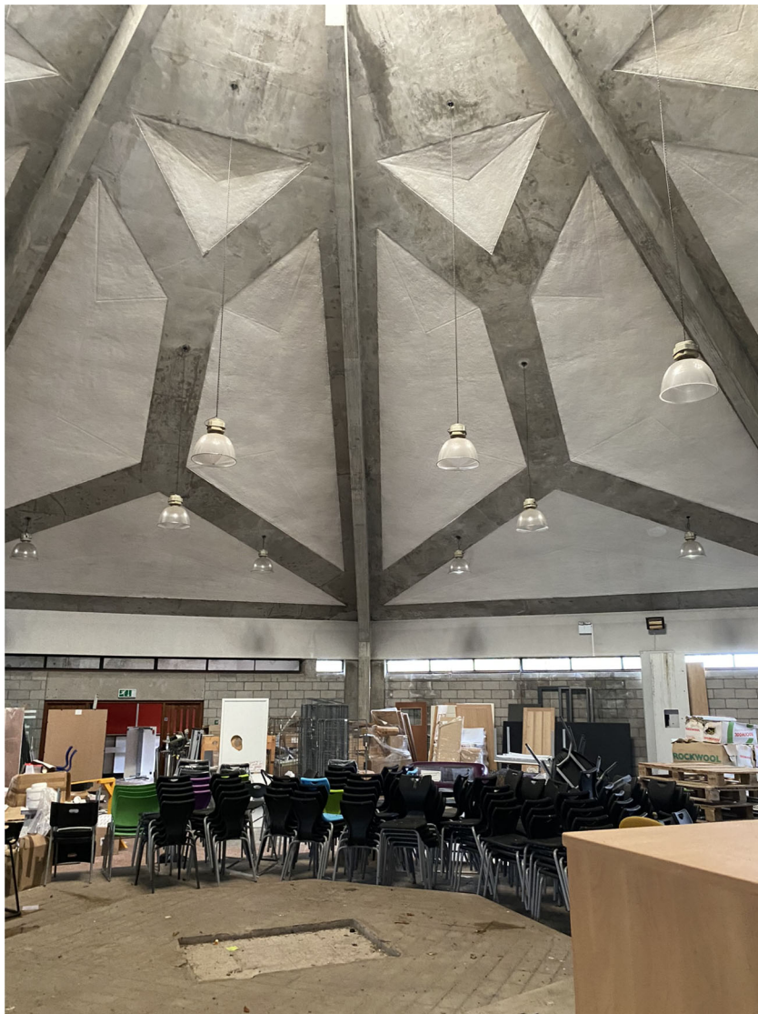
Interior View showing asbestos soffit and high level wall panels
