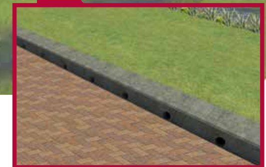
Marshall's Beany combined kerb and drainage into a swale
