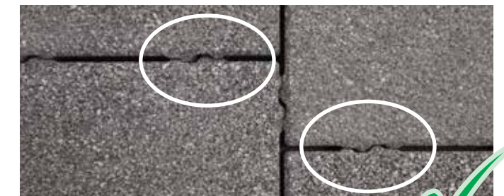
Correctly interlocking nibs
