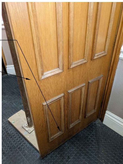
EXISTING VIEW OF DOOR FROM G10b (LOBBY) SIDE
