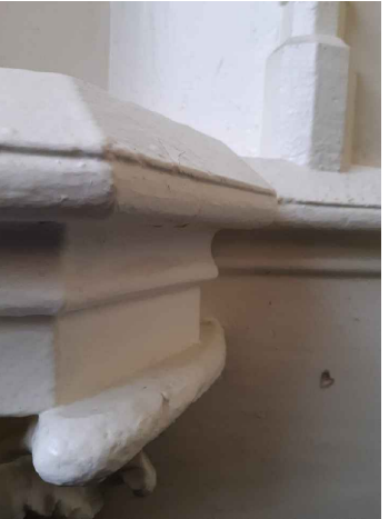
IMAGE 4 - String course detail runs around corbel base.
