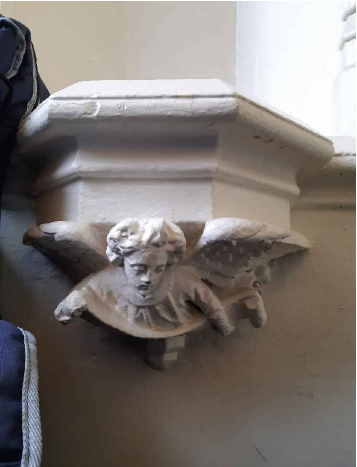
IMAGE 3 - Angel stone corbel at base of south east niche.
