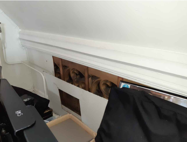
IMAGE 5 - Timber string course detail to west elevation and decorative eaves beam.
