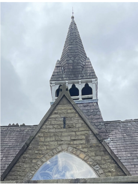
Cupola wooden structure undamaged; requires further inspection
