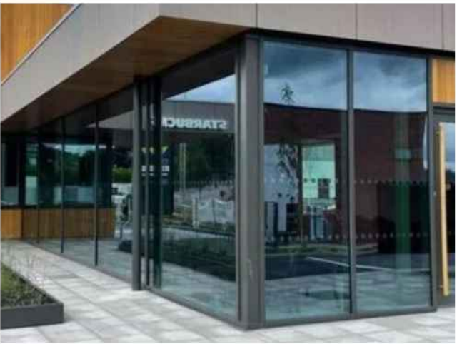
03. PPC aluminium full height curtain wall double glazed with manifestation - mullions RAL 7022 Umbra Grey finish
