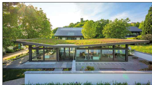
6. Sedum roof (inset)
