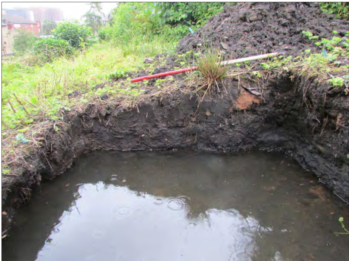
Plate 16: Test Pit 11 excavated as fully as possible prior to groundwater inundation
