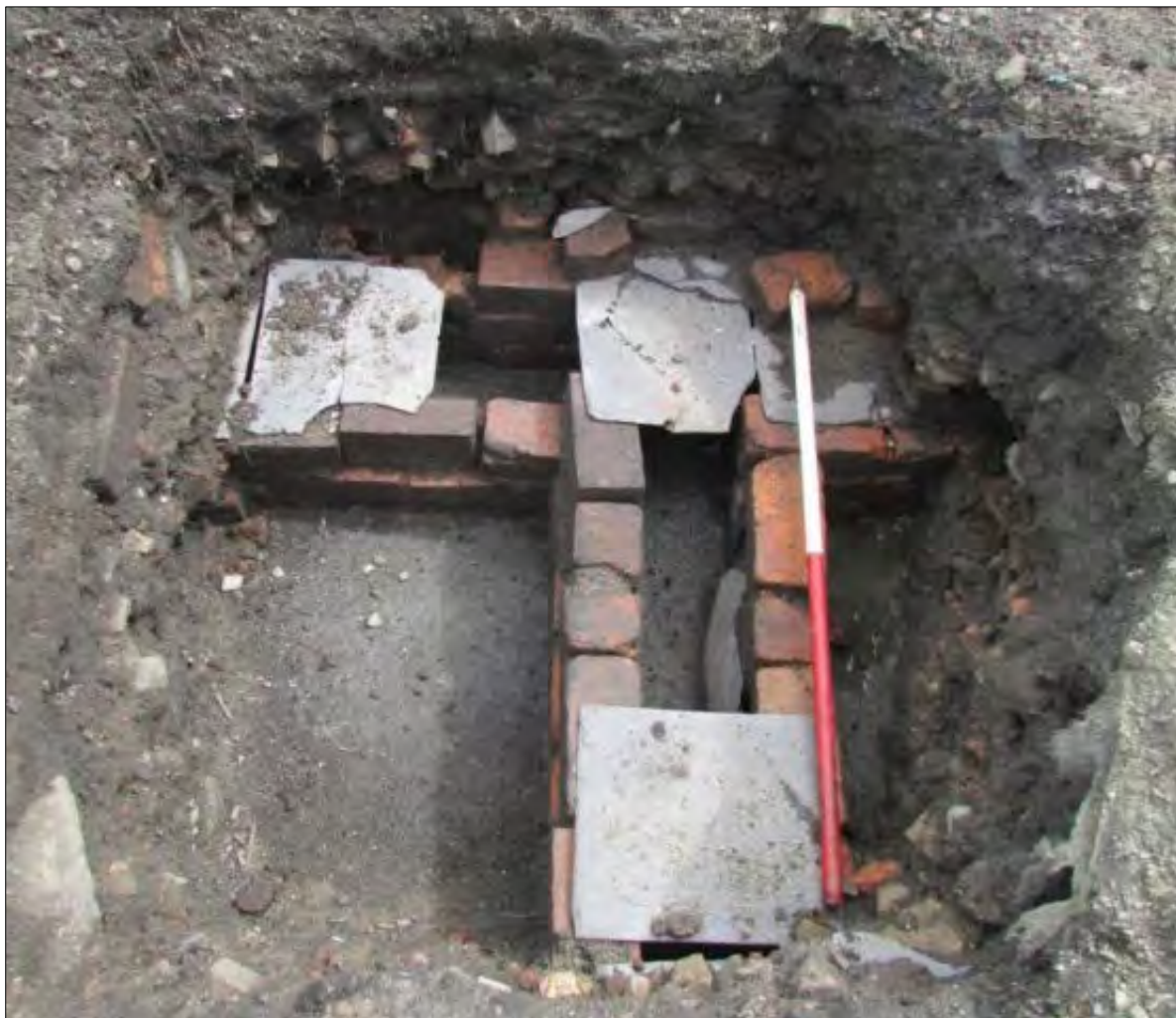
Plate 30: West-facing view of box drain 2402
