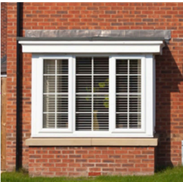
Modern Flat Roof Bay Windows
